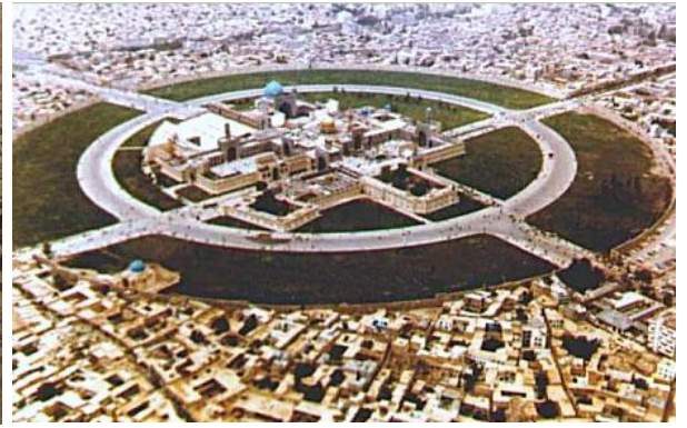
Shrine area after 1977. The shrine is still the most eye-catching building. However, the bazaars around the shrine are demolished and it has lost its relationship with the context. Photo taken by Georg Gerster, 22/09/77 (Gerster, 2009).
