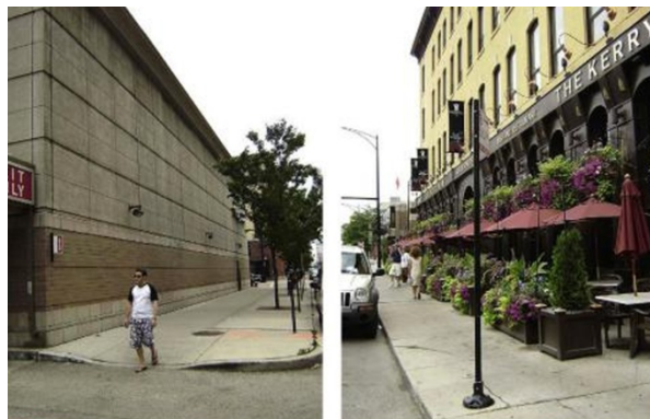
Figure 5: The impact of rigid walls, two sides of one street (Carmona et al., 2010:217).
