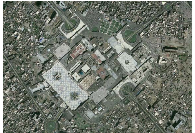
Shrine area in 2010. The shrine is almost lost in the large buildings which surround it (Google maps).
