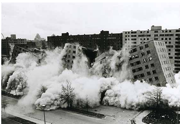
Figure 1: Pruitt-igoe Being torn down with a $300 Million loss (Newman, 1996b).
