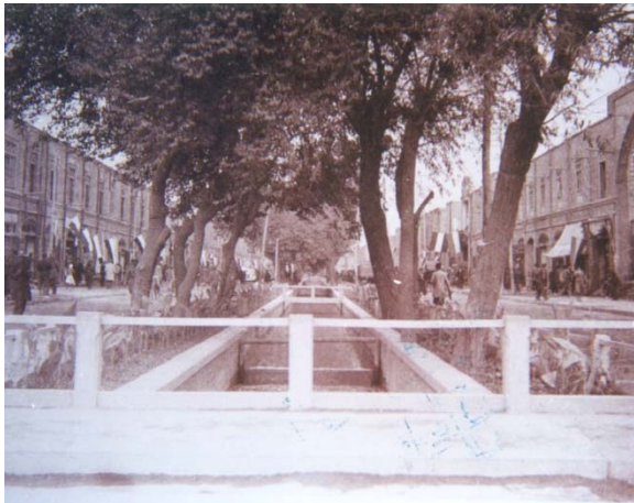
Bala-Khiaban in 1936-1941, the canal had concrete walls.
