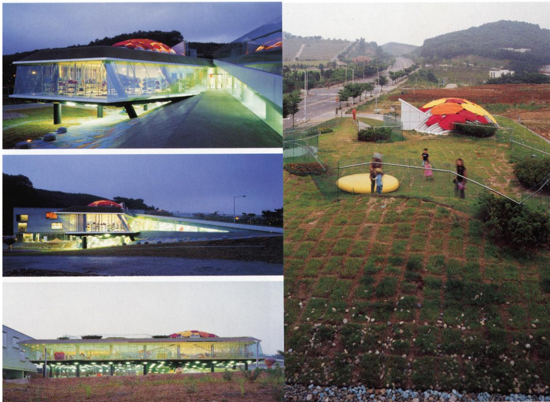
Figure 5.19: The roof garden. 194
