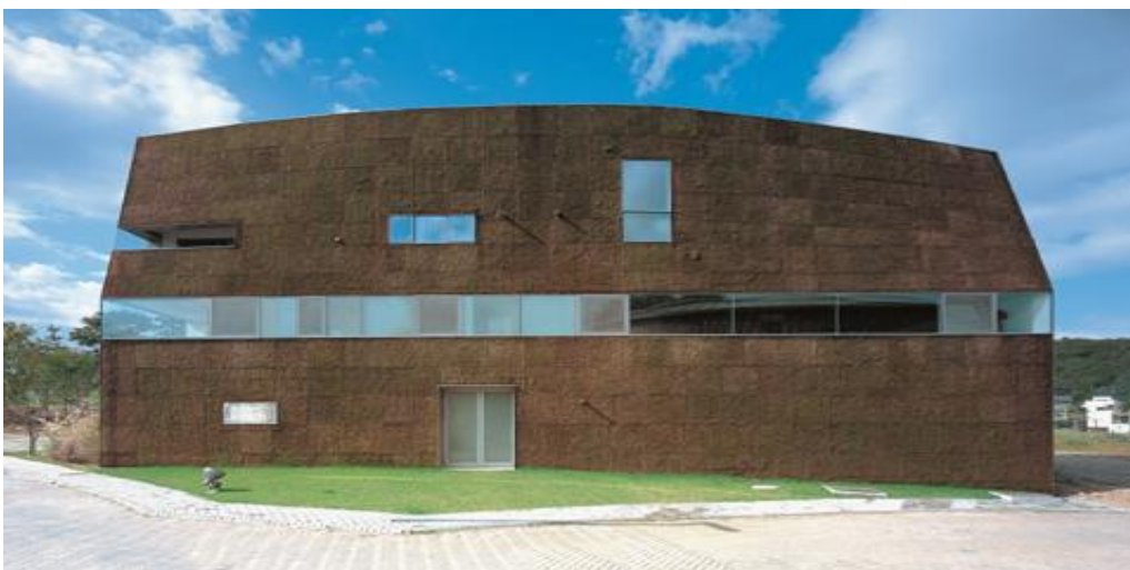
Figure 5.21: Torque House exterior.
