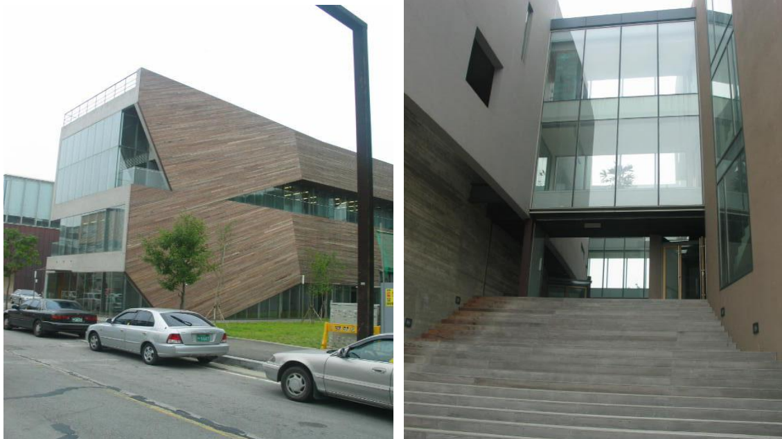
Figure 5.33: House of Open Books exterior and entrance.
