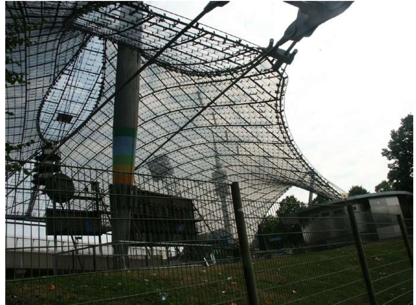
2.146 Interior of tent structure, Olympic Park (1972)
