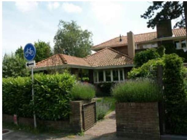
2.066 Front view, Simon Stevinweg Street (1923)
