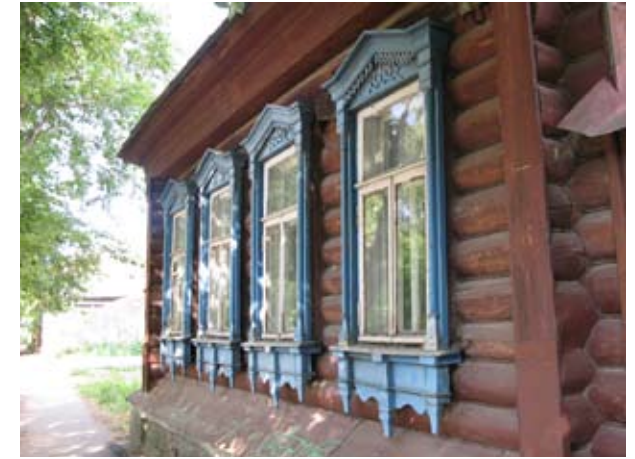
3.121 Timber construction to house, Egor'evsk
