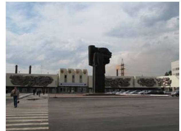
3.104 Entrance to the Steelworks
