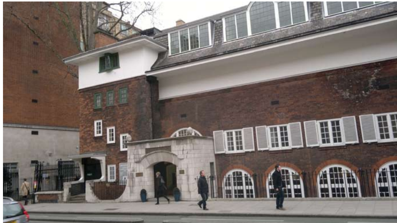
4.034 Street view of Mary Ward Settlement House with render band beneath the eaves
