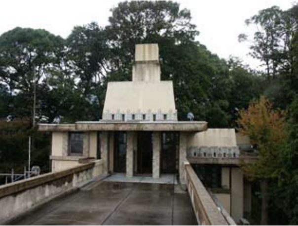
1.132 Third floor, external terrace, Yamamura Villa (1918)
