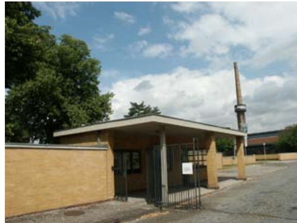
2.101 Entry pavilion, Fagus Factory (1911-12)
