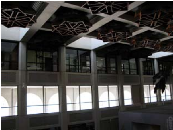
6.111 Ceiling detail to exhibition space within National Library and Cultural Centre (1978-81)
