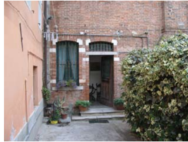
5.050 Common entrance door to apartment, Guidecca
