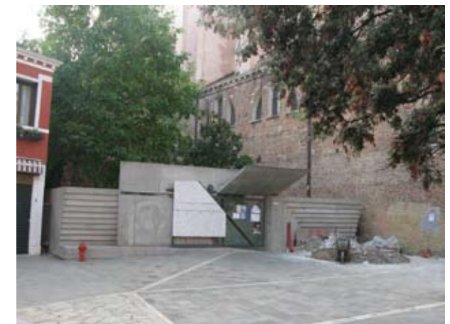
5.067 Entry to University Institute of Architecture (1966, 69, 72)
