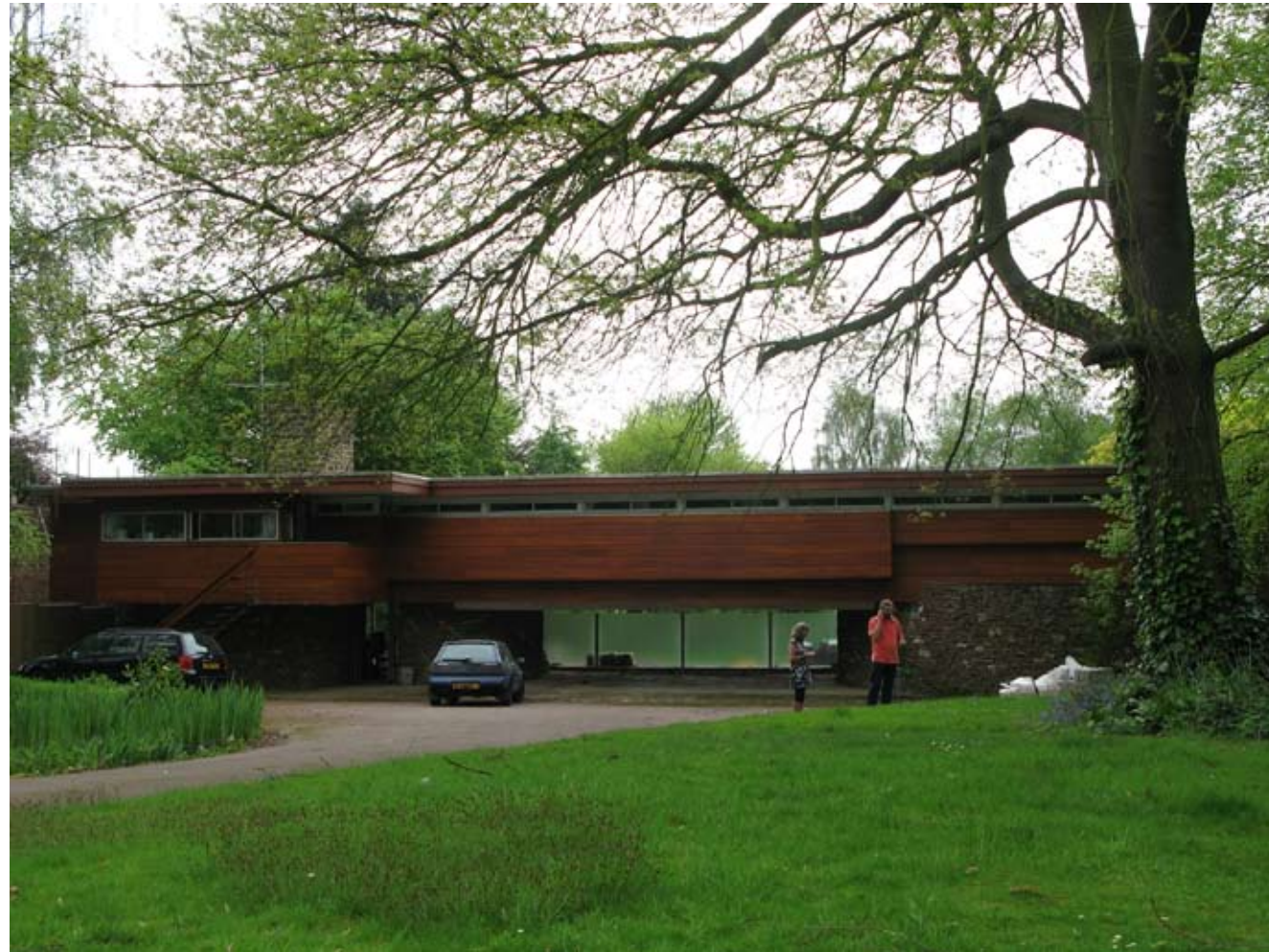
4.113 Rear view from the road to South Winds
