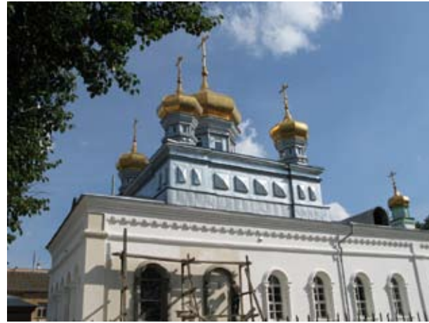
3.119 Restored church with stone base metal cladding above, Egor'evsk
