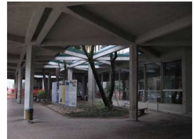
5.103 Undercroft to Social Services Building (1954-7)
