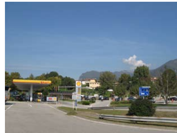
5.028 Service station, Lugano, Switzerland
