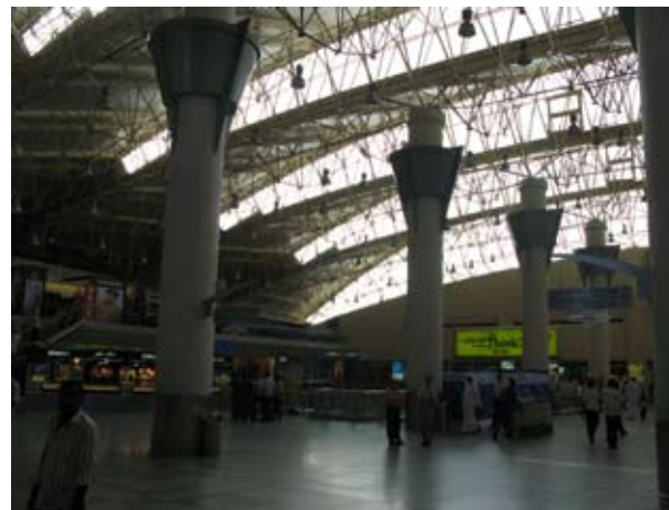
6.025 Departures, hall at Kuwait International Airport
