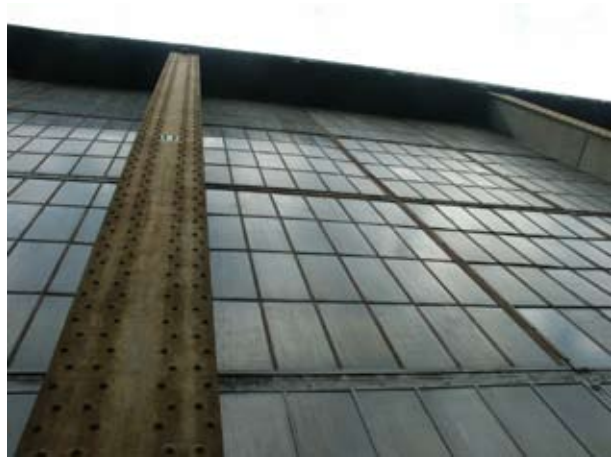
2.100 Side column, AEG Turbine Factory (1908-09)
