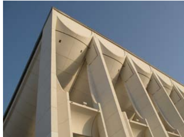
6.055 Entry Canopy detail to National Assembly Building (1985) by Jorn Utzon
