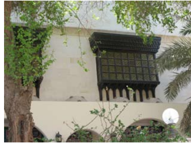
6.068 Screened window detail to Tareq Rajab Museum Villa
