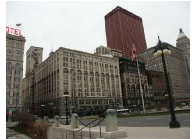
5.118 Street view of Auditorium Building (1887-89)
