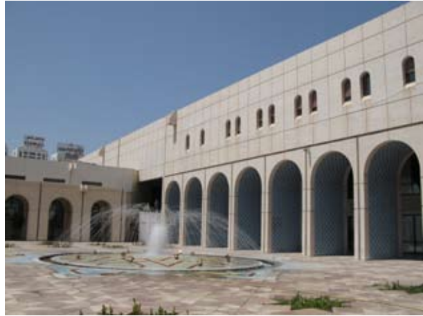
6.109 Internal courtyard to National Library and Cultural Centre (1978-81)
