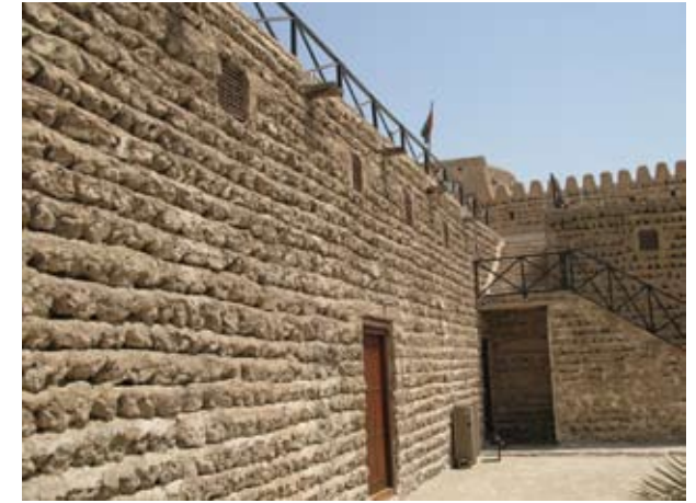
6.085 Defensive wall to Dubai Fort
