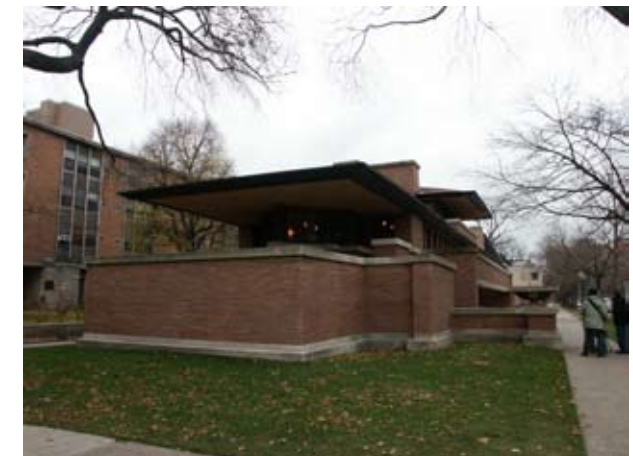
3.129 View 2. Corner Terrace, Robie House
