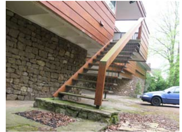
4.114 Stairs leading to first floor kitchen, South Winds
