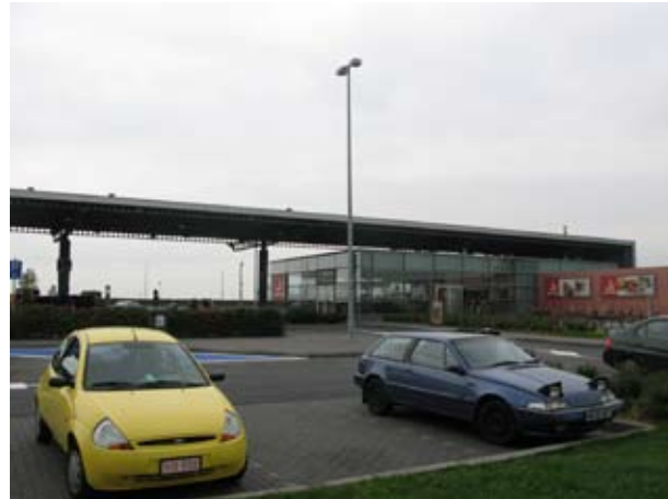
5.022 Service station, Brugge, Belgium
