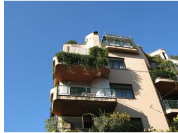
5.135 Corner balcony to Palzzoino (1952)
