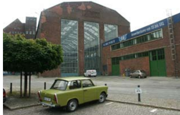
2.093 External view, Assembly Hall for Large Machines (1911-12) by Peter Behrens
