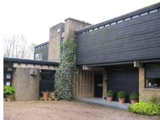
4.129 Rear view and entrance, Clayton House (1965-6) by Aldington and Craig
