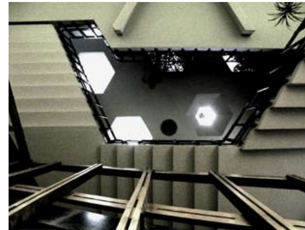
5.106 Internal stair to Social Services Building (1954-7) When Frank met Francesco
