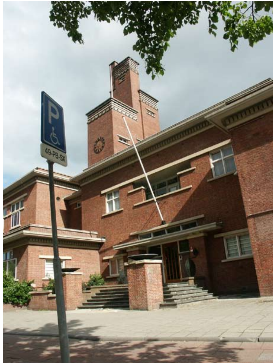
2.033 Street view, Sint Franciscus College, Secondary School (1922-4) by H. Sutterland, and P. G. Buskens.
