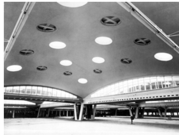
4.089 Production hall (1951), image from (RIBA2832-23) Whatever Happened to Frank Lloyd Wright
