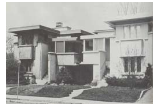
4.044 Street view of 'Two-Family-Flat-C' Duplex Apartments Arthur L. Richards (1916), Milwaukee, WI, which appears on page 118 of said book; image from Meehan, Patrick J. (c) 1987, 1992, and 2014. Copyright (c) Patrick Joseph Meehan, 1987, 1992, and 2014. ALL RIGHTS RESERVED.
