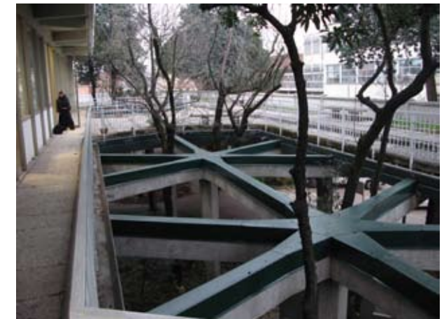
5.107 Openings in the terrace for trees to project Social Services Building (1954-7)
