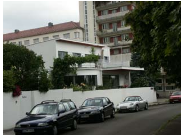
2.130 Exterior view, House 33 (1927) by Hans Scharoun
