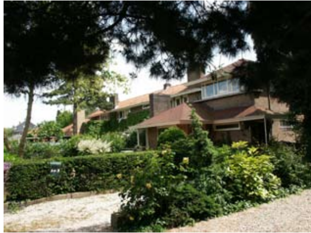
2.063 Garden view, Simon Stevinweg Street (1923)
