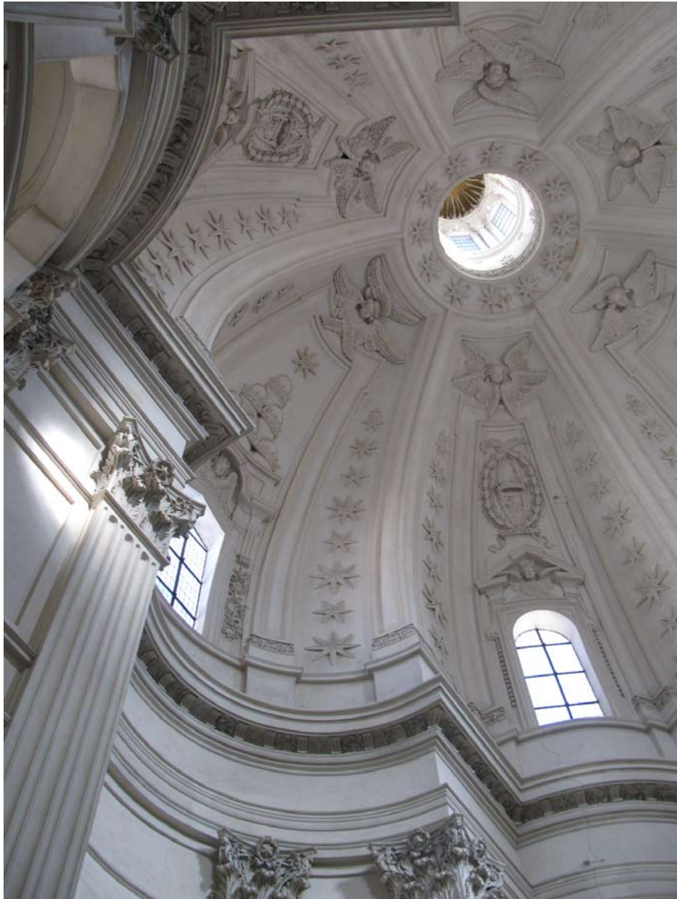
5.178 Interior view of ceiling with two intersecting triangles generating a hexagonal module within St Ivo della Sapienza (1642-60) by Borromini
