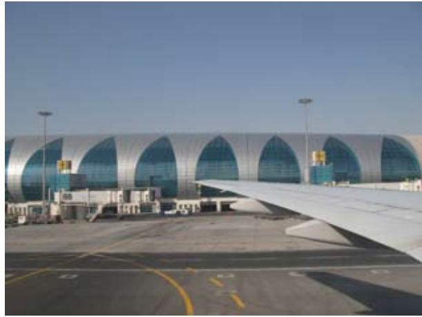
6.077 External view from plane of Terminal 3, (2008) Dubai Airport
