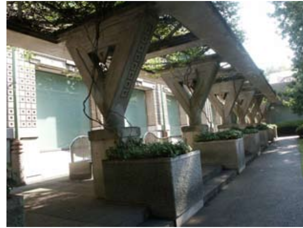
1.205 External pergola, triangular forms from Wright's drafting room at Taliesin North, Setagaya Museum (1985)
