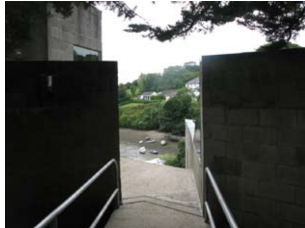
4.134 Bridge from the road, entrance door to the left, Creek Vean (1963-6) by Team 4
