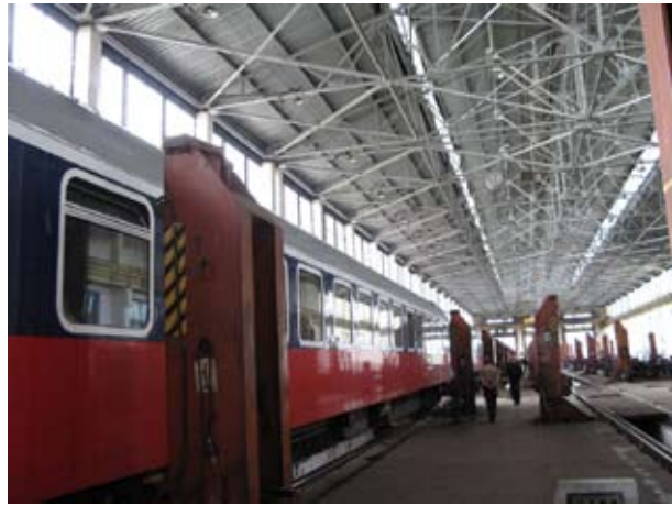
3.011 Preparing to lift the train carriages, train shed, Poland / Belarus
