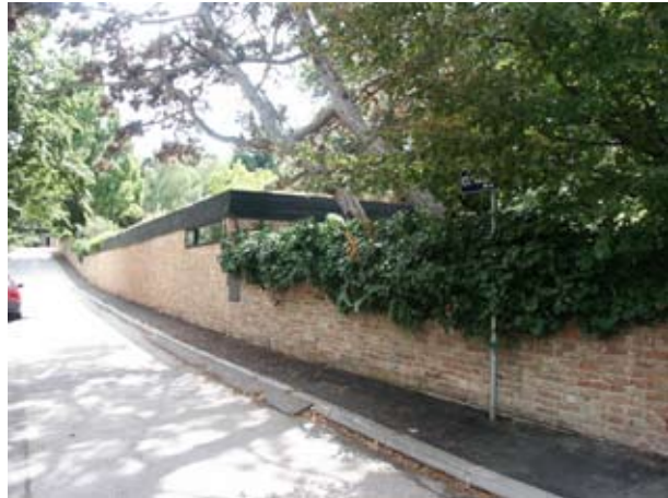
2.153 Perimeter wall to Haus am Nordhang and Haus unter Baumen (1968) by Ronald Rainer
