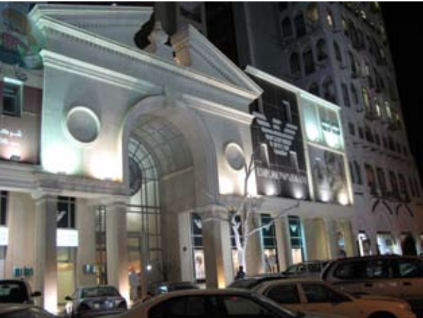
6.049 Street view of Central Mall
