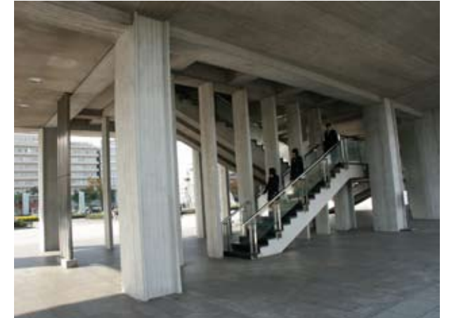
1.184 Entrance, Hiroshima Peace Centre Complex (1949-52)
