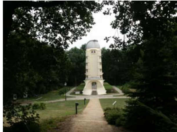
2.107 External view, Einsteinturm (1921) by Medelshohn
