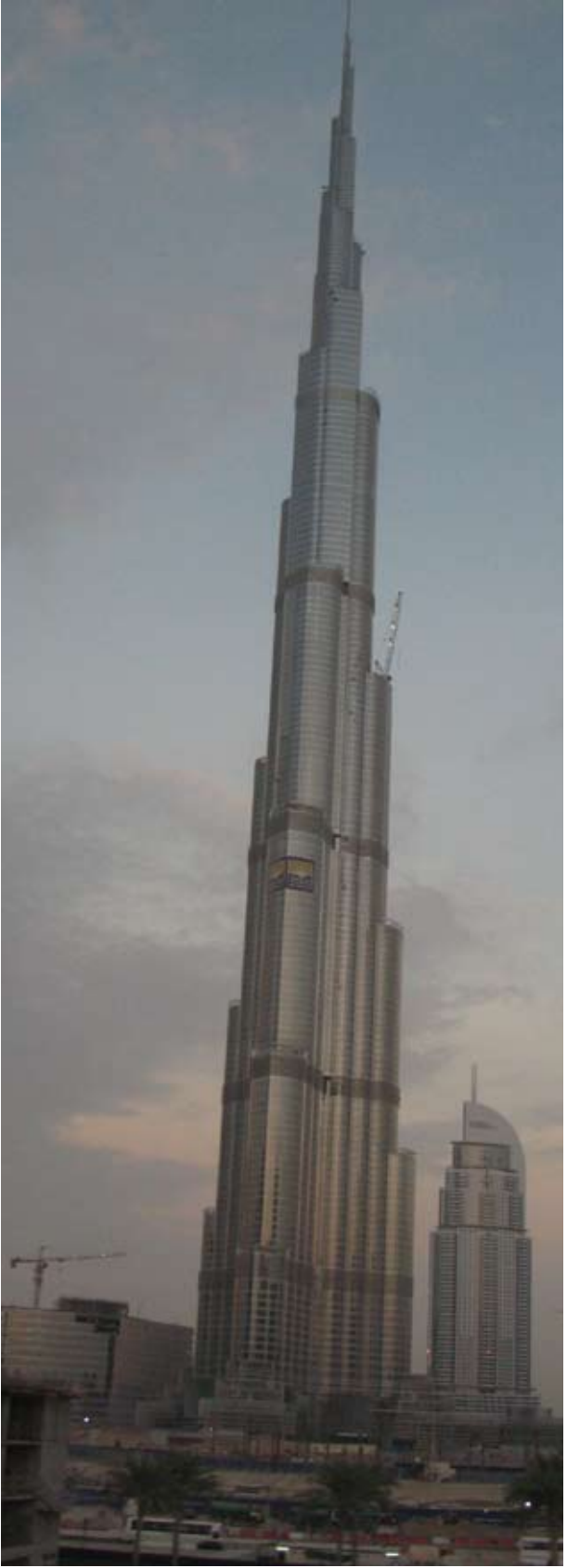
6.102 View of Burj Khalifa Tower (2010) by SOM, Chicago
