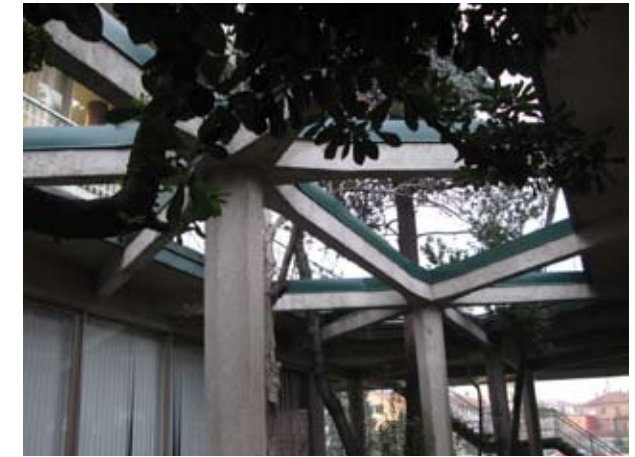
5.105 Openings in the terrace for trees to project Social Services Building (1954-7)
