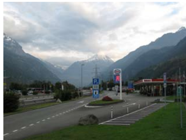
5.027 Service station, Aldorf, Switzerland
