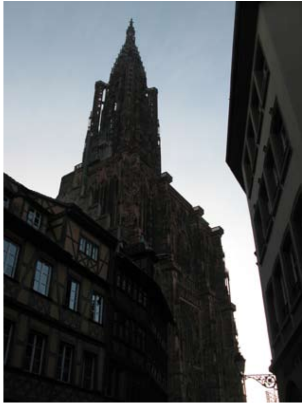
5.173 Exterior view of Strasbourg Cathedral, France (1176-1439)
