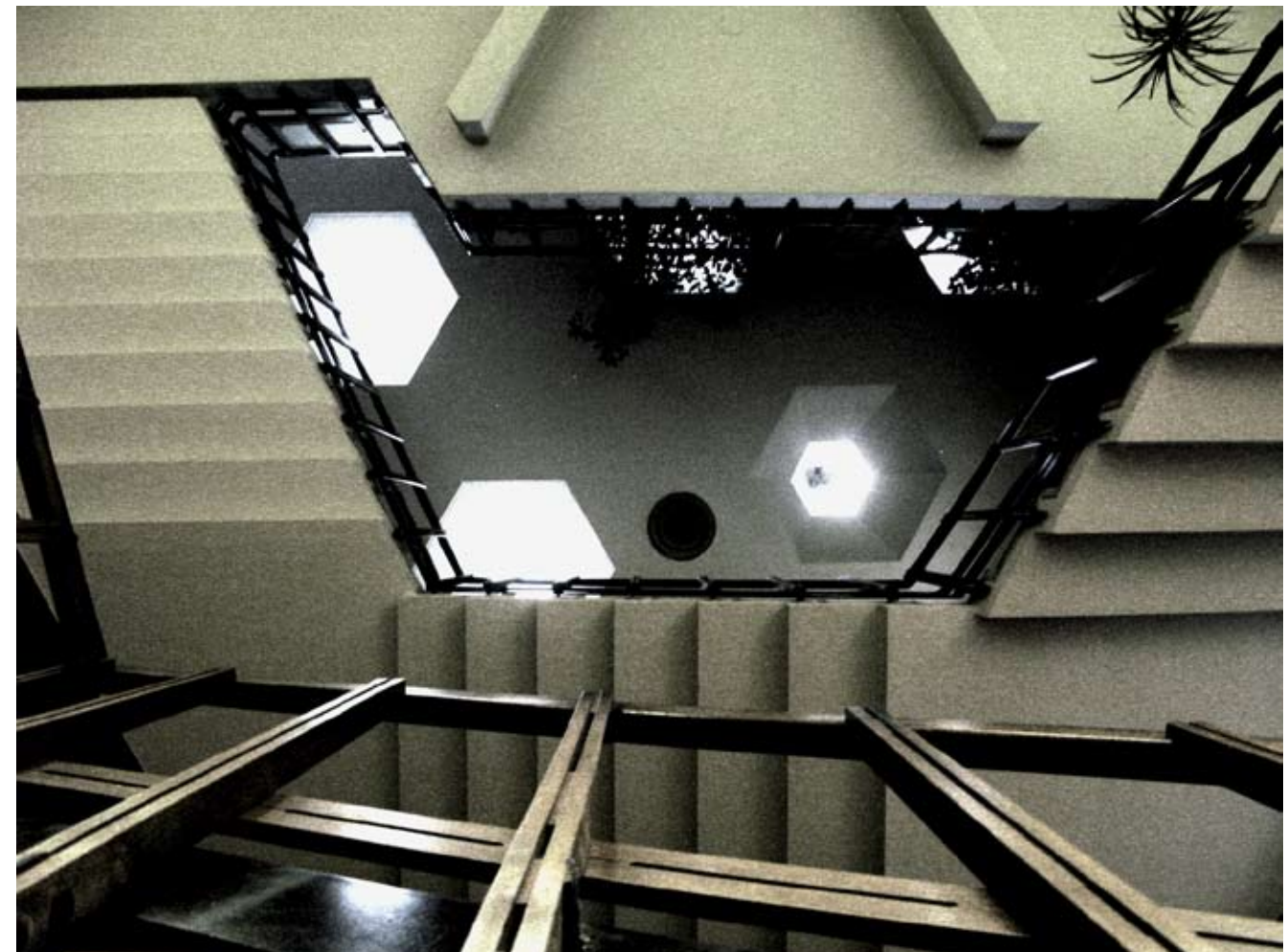
5.179 Interior view of hexagonal skylights to Olivetti Social Services Building (1952) by Figini and Pollini
