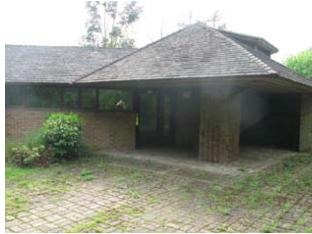
4.099 Corner entrance, Number 112 and 114 Kenilworth Road.
