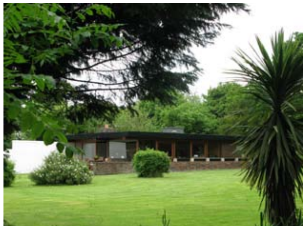
4.131 Garden view, Long Wall (1963) by Dawson and Foggo
