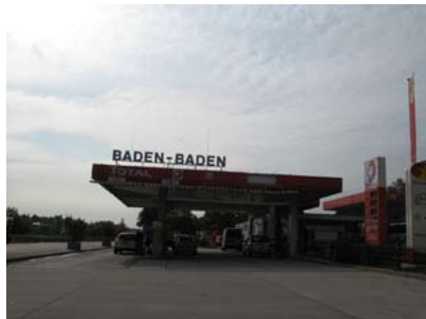
5.026 Service Station, Baden - Baden, Germany
