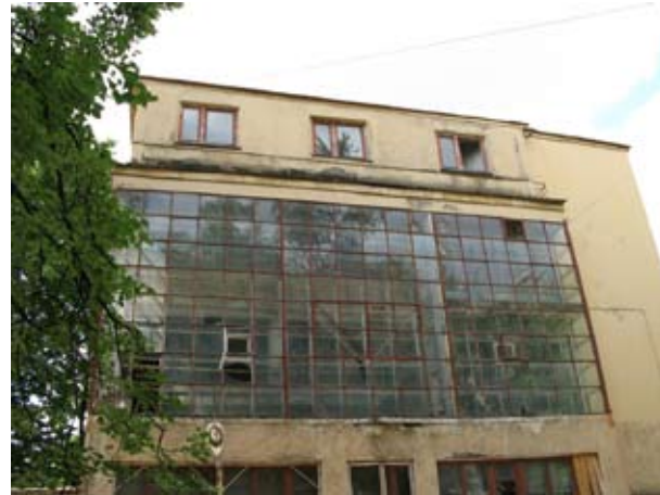
3.026 Exterior view of communal unit, Narkomfin Housing Complex (1929)
