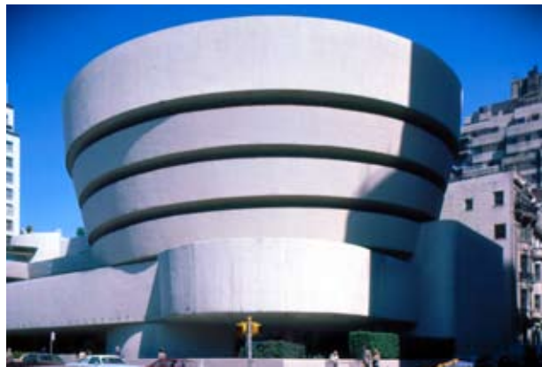
5.167 Exterior of Guggenheim Museum (1946-59) by Wright, photograph by Bernard Cox (RIBA3072-36)
