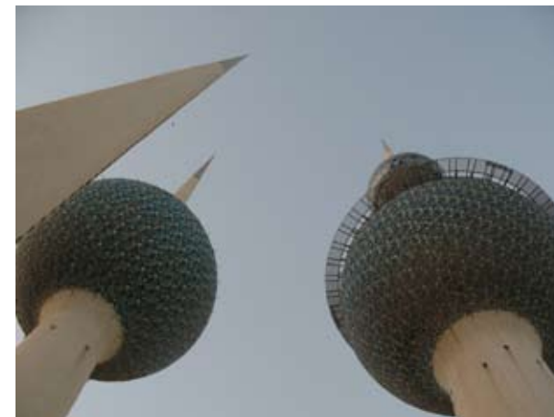
6.063 View looking upwards of the Water Towers (1979)
