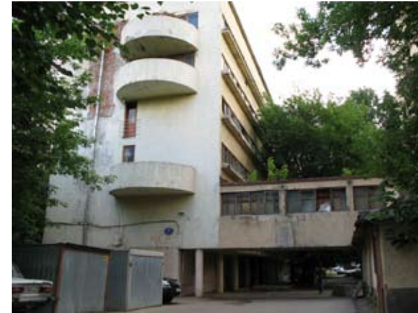
3.027 End view of housing unit, Narkomfin Housing Complex (1929)
