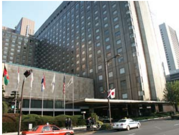
1.046 Street view of entry (2005)
