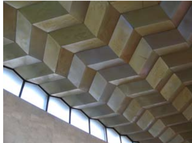
3.137 Ceiling detail of Leningradsky Railway Station Moscow
