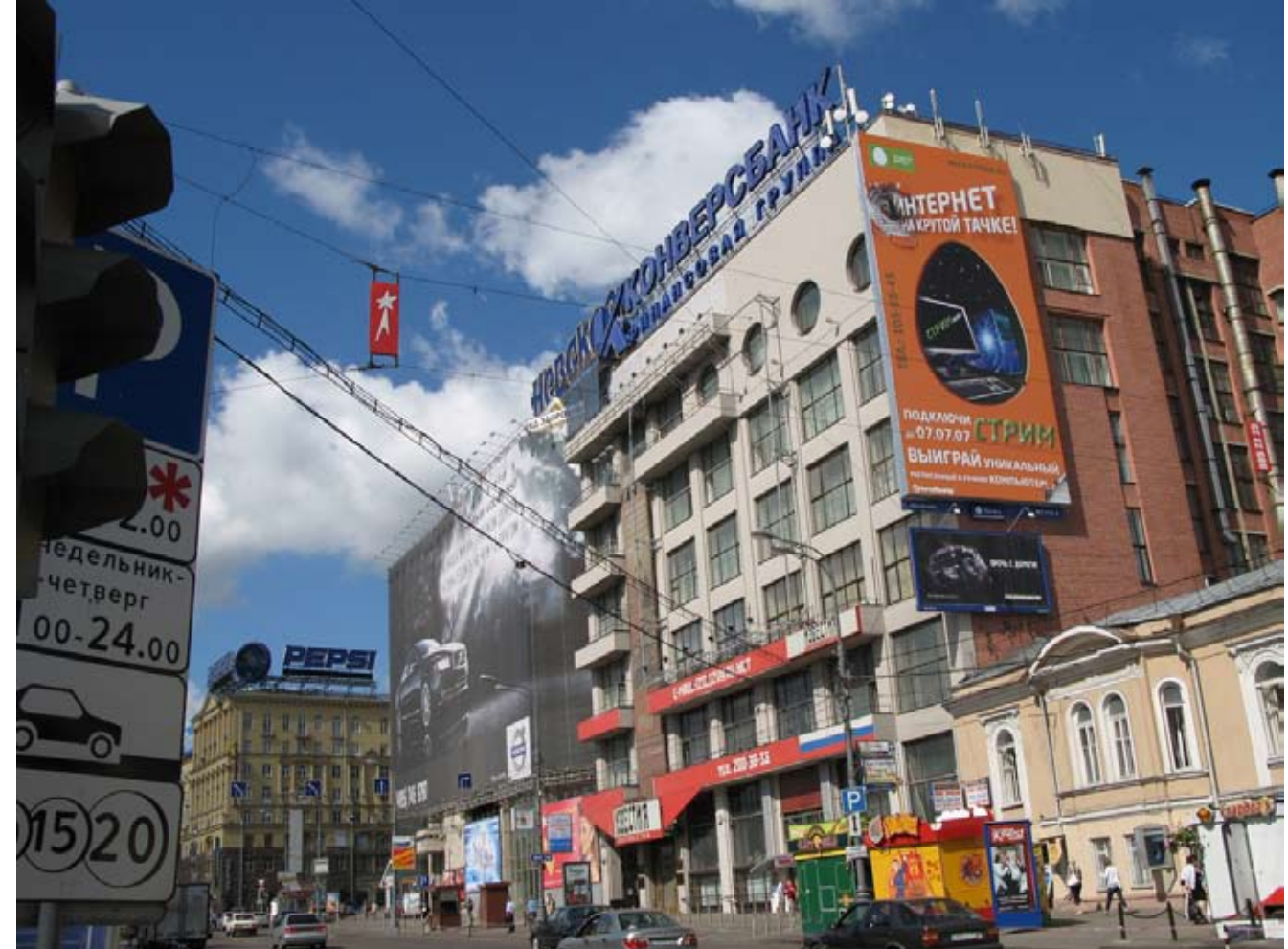
3.024 Exterior view, Isvetsia Building (1925-7) by Barkhin
