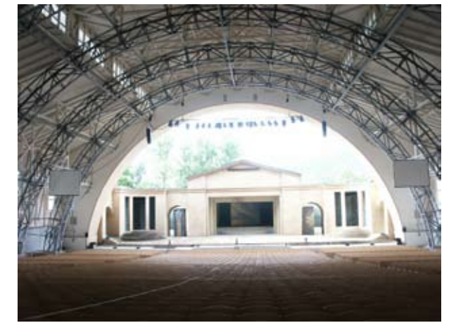
2.151 Interior view, Obermergau Opera enclosure
