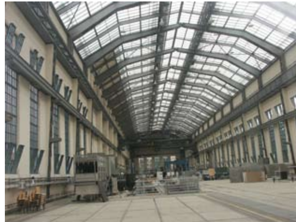
2.094 Interior view, Assembly Hall for Large Machines (1911-12)
