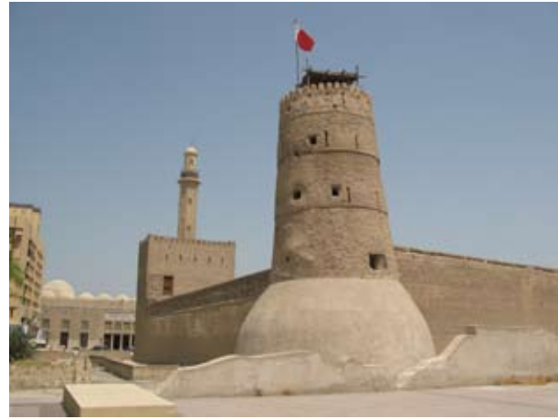
6.083 Exterior view of Dubai Fort with Dubai Museum beneath
