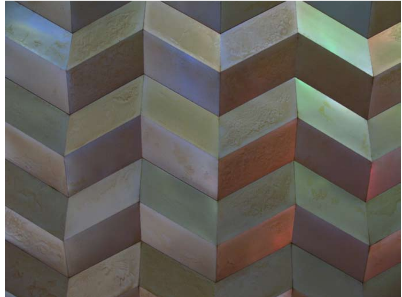
3.138 Ceiling detail of Leningradsky Railway Station Moscow
