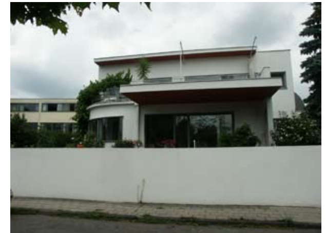
2.132 Perimeter wall with living space behind, House 33 (1927)
