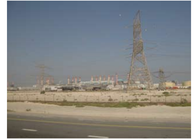
6.106 Power station in the desert
