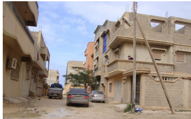
Photo 6. 15: Building Type, Site Four - El-Salam-I Vertical intensification Source: Own photo, 2010
