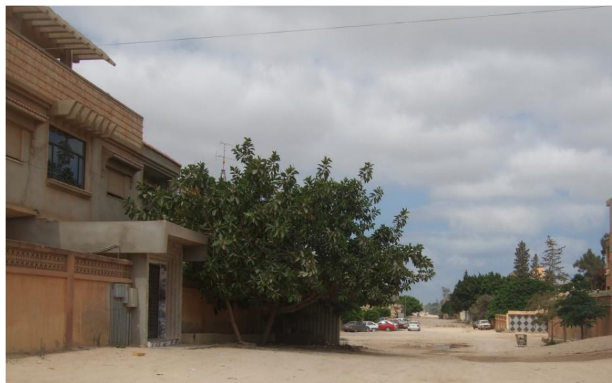
Photo 6. 24: Detached Building, Site Seven - El-Mukhtar-B Area
