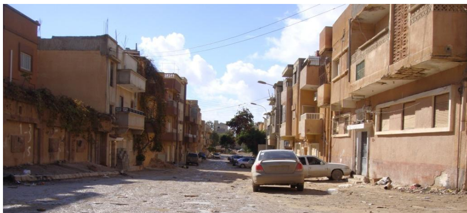
Photo 6. 20: Street View, Site Five - El-New-Benghazi Area
