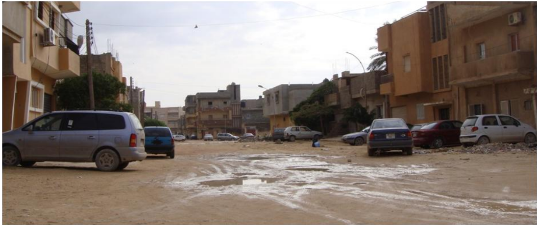
Photo 6. 13: Residential Street, Site Four - El-Salam-I
