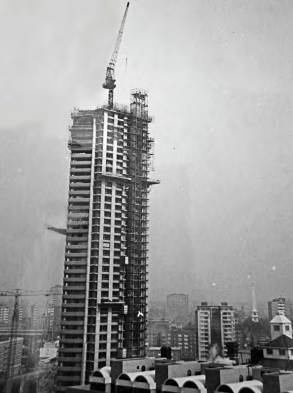
Barbican tower under construction Source: Courtesy of Richard Organ
