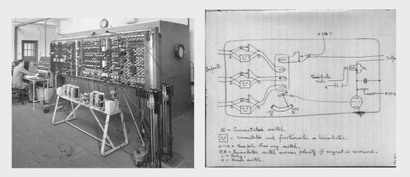
Fig. 4.18 The NPL (National Physical Laboratory) ACE Pilot computer designed by Alan Turing, 1945-50
