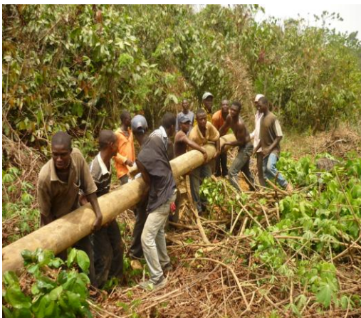
Farmers Erecting an Electric Pole (Rural Village) 03/03/09
