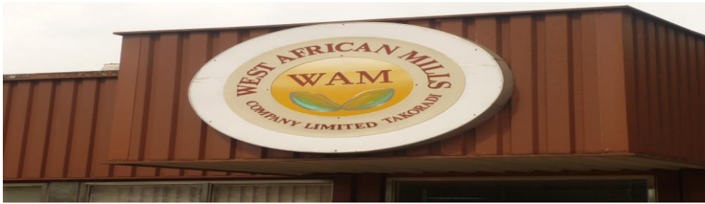
Figure 5.5 WAMCO Factory after the Refurbishment
