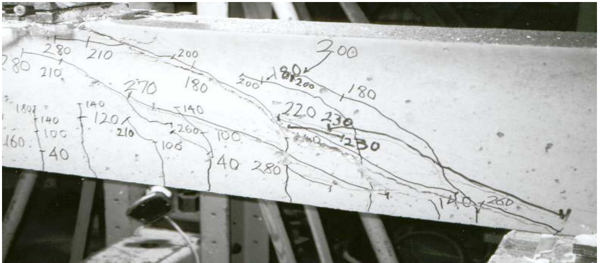
Figure 3.15: High Strength Beam (HSC4) with the angle of crack at about 42°
