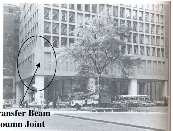
Figure 6.2: External TBCJ at Brunswick building, Chicago, USA
