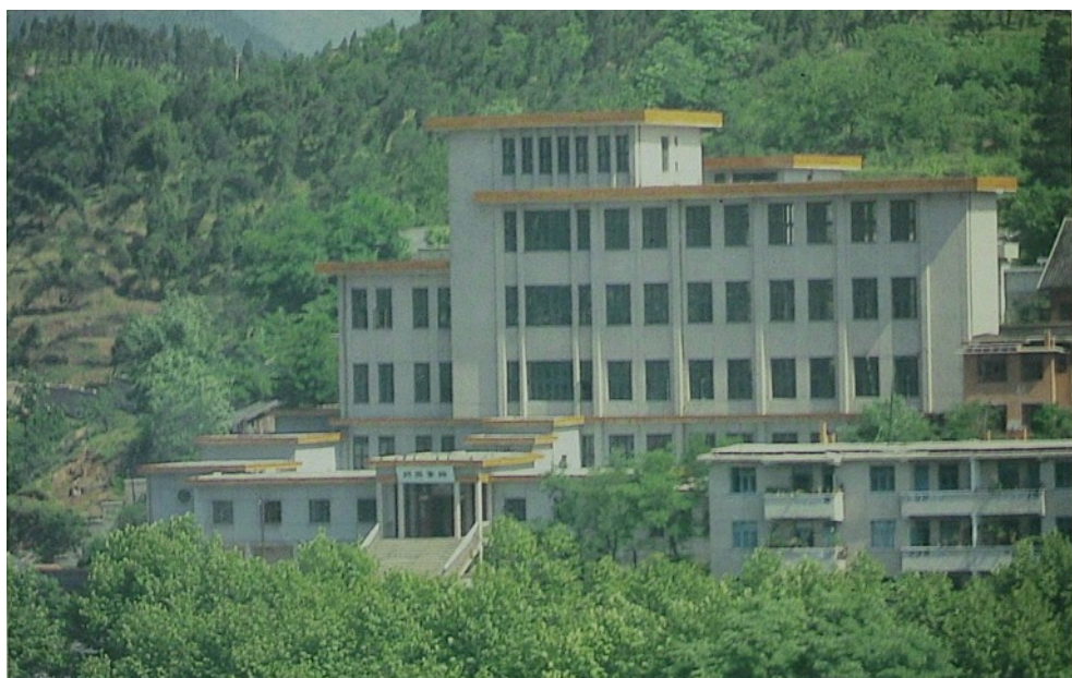
Figure 5.2: The prefectural library demolished to facilitate the park entrance (Xiong 1998)
