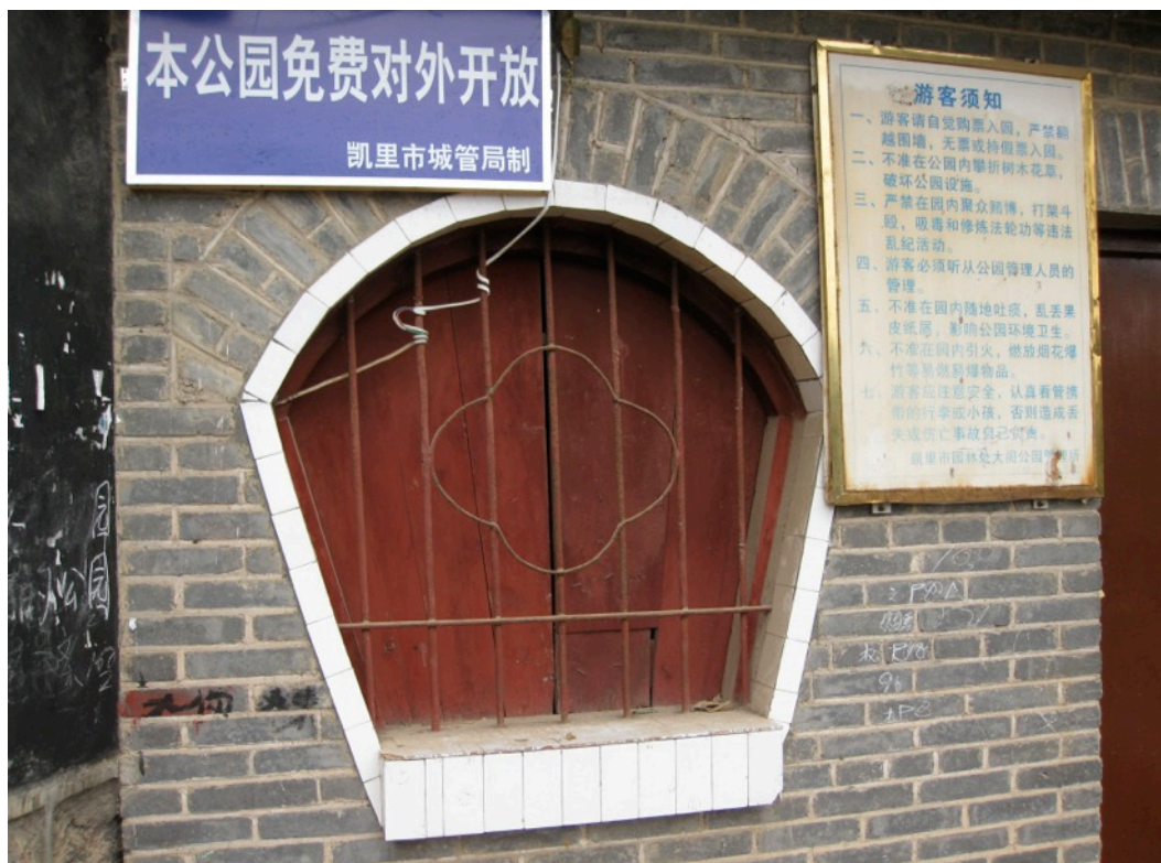
Figure 5.3: Abandoned ticket booth in Dage Park. Blue sign (top-left) reads: “This park is free and open to the public” (fieldwork photo 2011)
