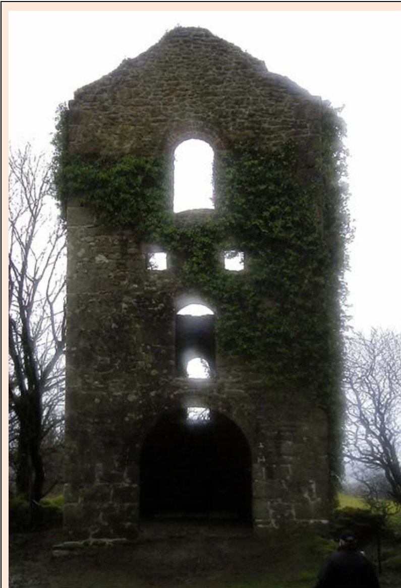
Figure vii. South Caradon Mine stabilisation
