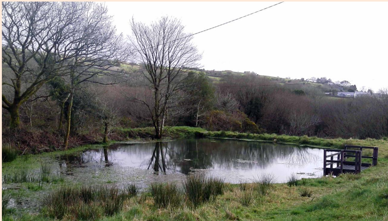
Figure vi. Toyz Pond restoration at Higher Tremarcombe
