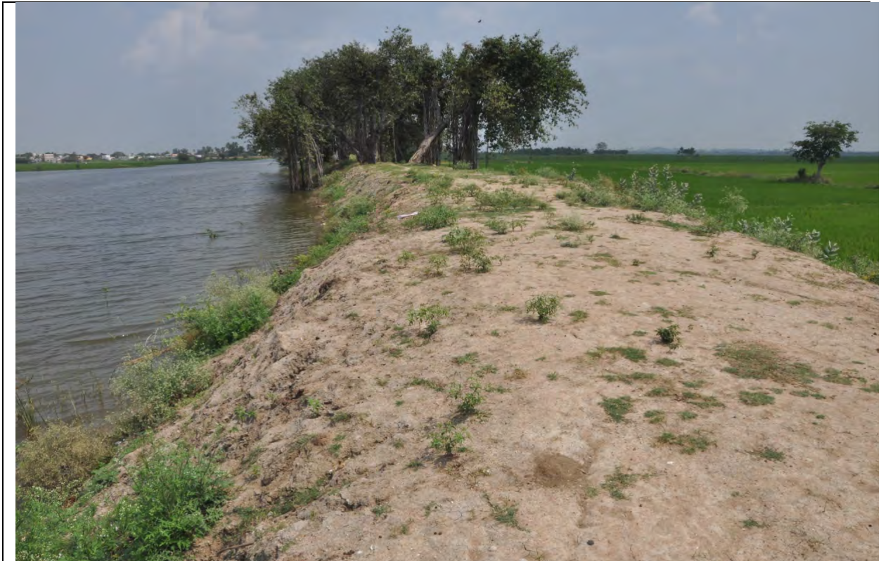
Photo 1 View of a Tank with water and Ayacut
