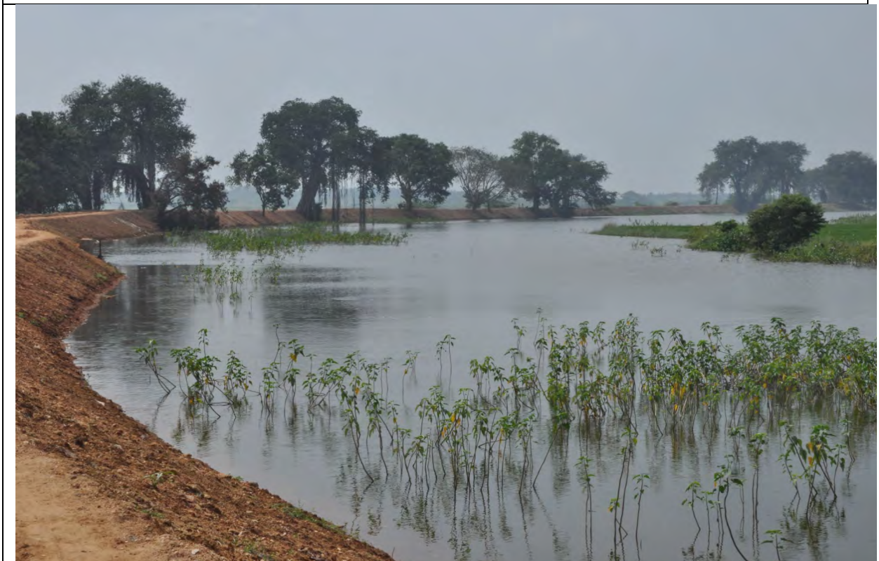
Photo 2 View of a Tank with water
