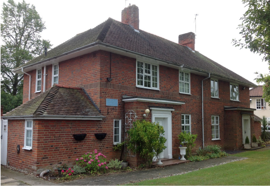
Howard's house at Welwyn Garden City: the semi-detached remains one of the most popular housing types in England (photograph by author; 2015).
