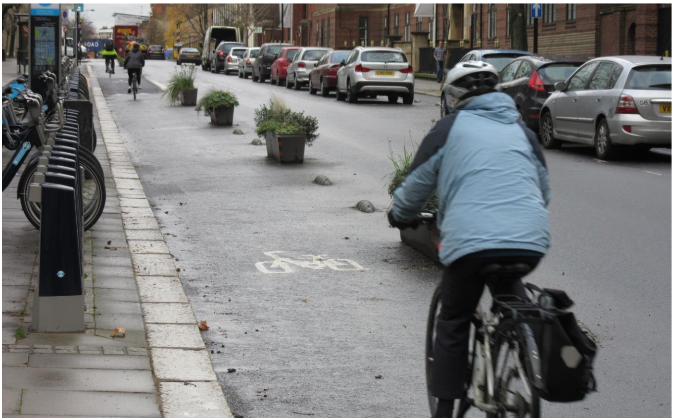
Figure 3: Royal College Street northbound track, separated by planters and 'armadillos', approaching one of the two bus stops
