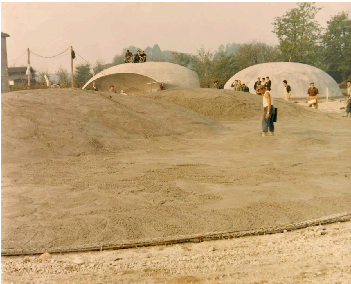
Figure 3. Castelfranco Emilia, Italy. Architect, Dante Bini. The first 30 metre diameter Binishell during inflation, 1967. Private archives of Dante Bini.
