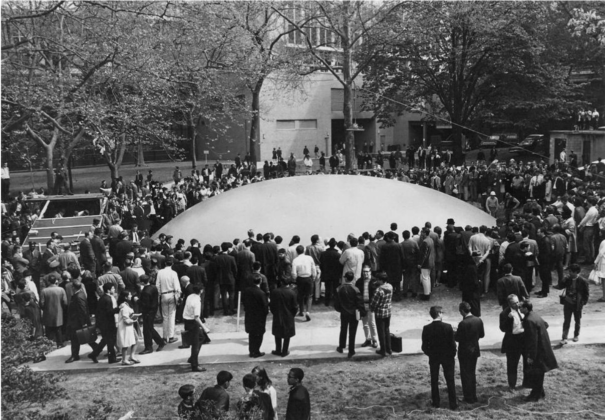
Figure 6. New York City. Architect, Dante Bini. Demonstration construction of a 15 metre diameter Binishell at Columbia University at the invitation of Mario Salvadori, 1967. Private archives of Dante Bini.
