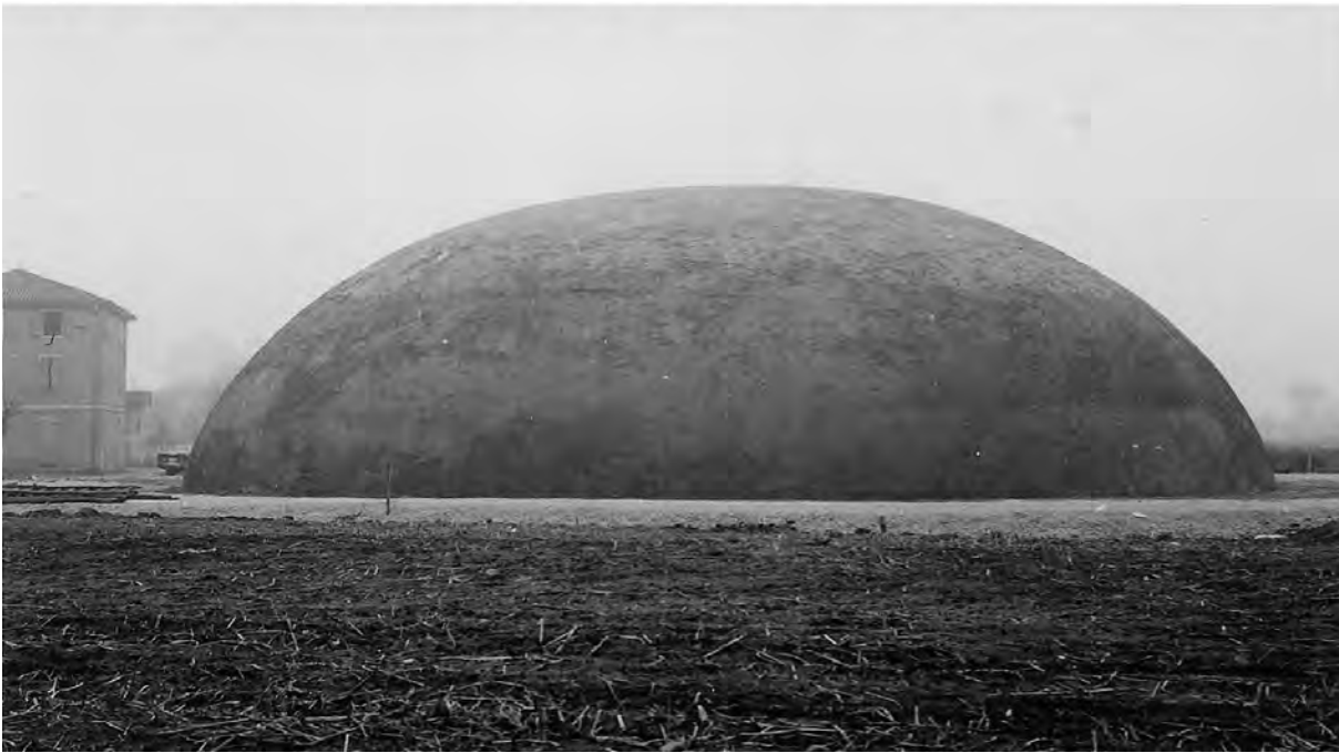
Figure 4. Castelfranco Emilia, Italy. Architect, Dante Bini. The first 30 metre diameter Binishell before and after construction, 1967. Private archives of Dante Bini.
