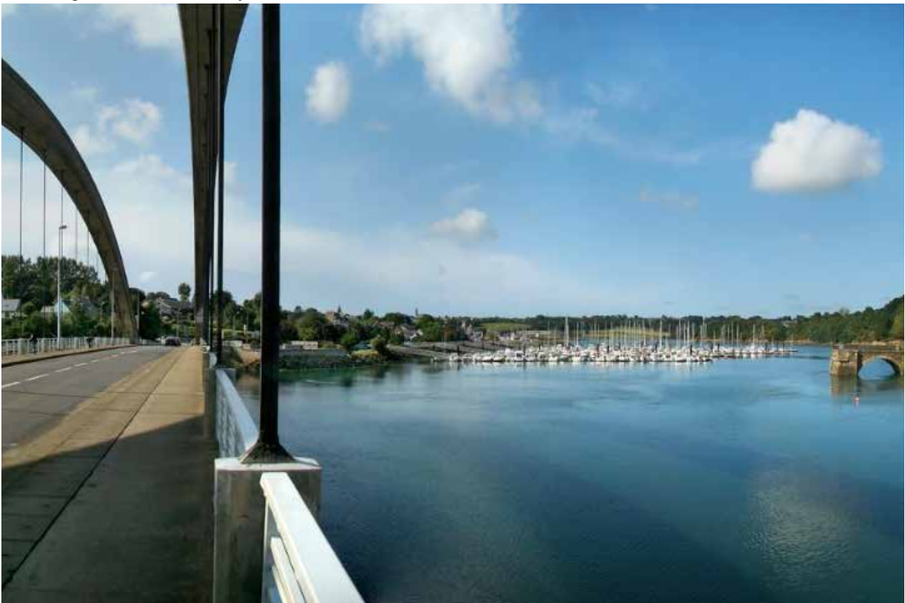
The bridge across the Jaudy river
