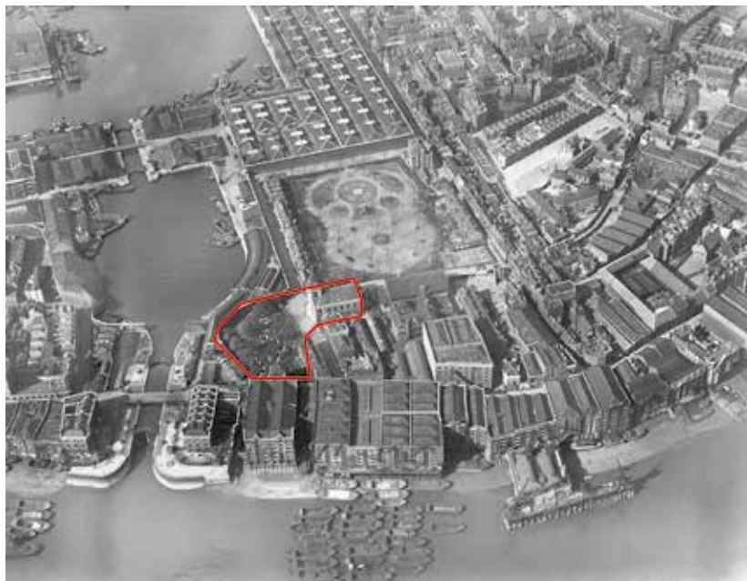
Figure 7.1. St. John's churchyard, Wapping, from the air, 1922. Photo: Historic England/britainfromabove.org.uk.
