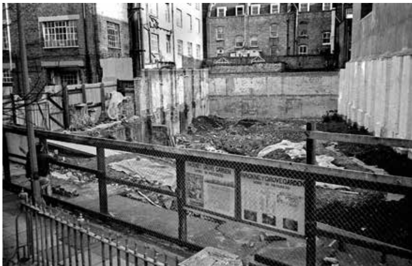
Figure 7.9. Hackney Grove Gardens 'Work in Progress', Jan. 1983. Photo: Alan Denney via flickr.
