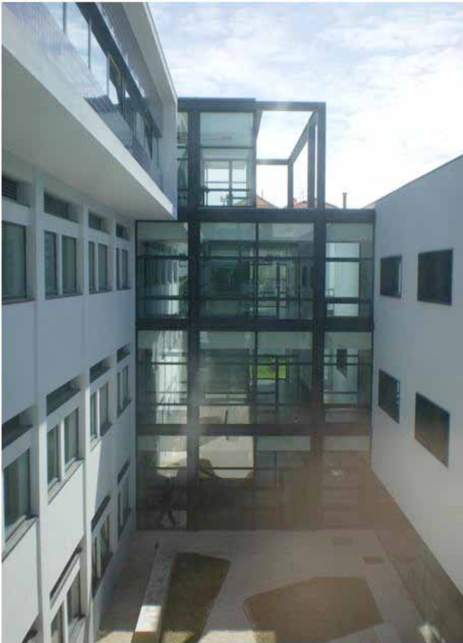
Figure 3.7. Connecting existing teaching blocks, Soares dos Reis Arts School, Porto
