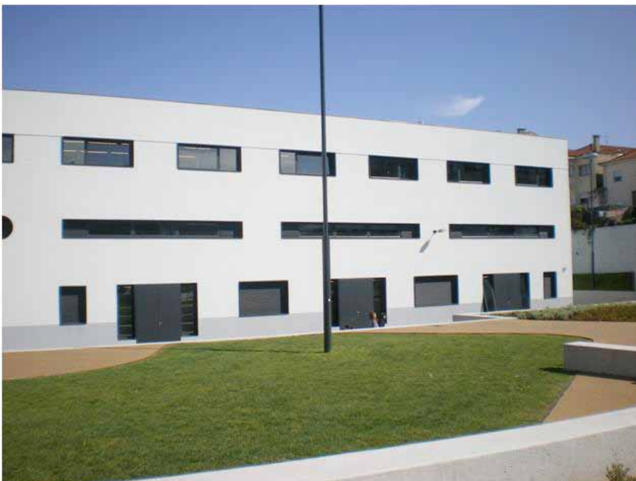
Figure 3.11. Facade, Soares dos Reis Arts School, Porto
