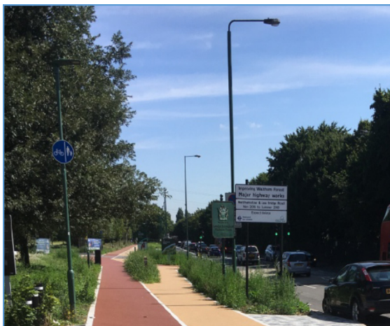
Fig. 2. New cycling infrastructure on Lea Bridge Road (photo: Joseph Croft, 2017).
