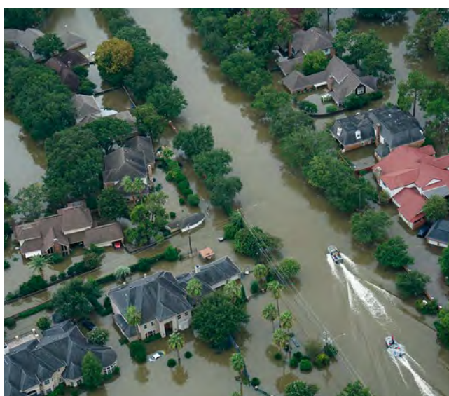
Flooded neighbourhood in the US after Hurricane Harvey in 2017
