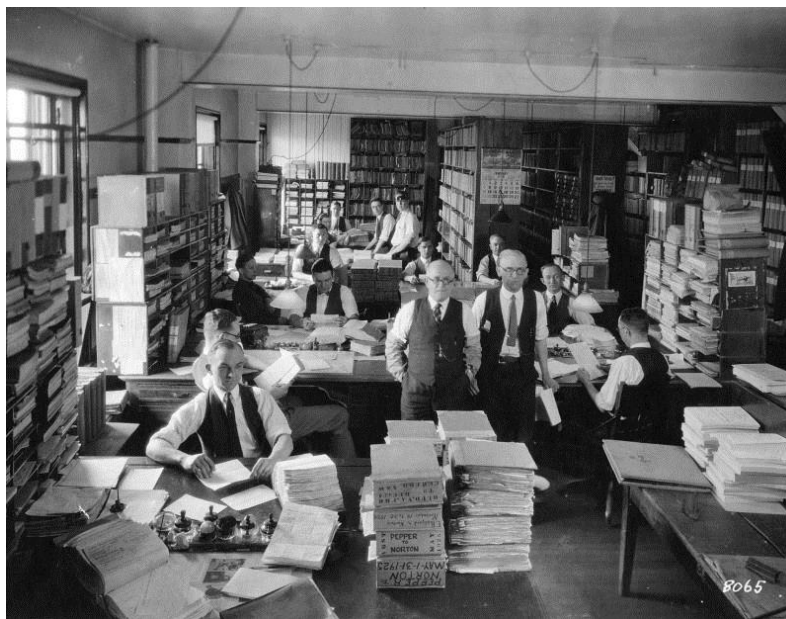
Figure 16 General office 1920s, Norfolk & Western Railway, Roanoke, VA. Norfolk and Western Historical Photograph Collection, Norfolk Southern Archives, Norfolk, Va., Digital image courtesy of Special Collections, Virginia Tech, Blacksburg, Va.
