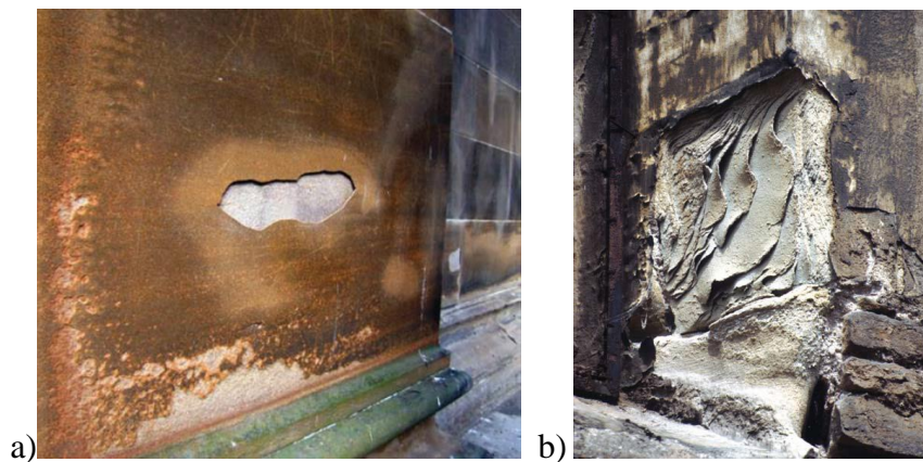
Figure 9. Detachment pattern: a) Blistering of sandstone (image: ICOMOS Glossary); b) Exfoliation of sandstone ( image: ICOMOS Glossary).
