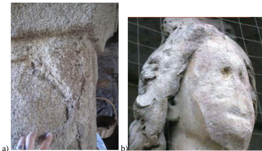
Figure 11. Powdering pattern: a) disintegration due to salt crystallisation of a column at the Pazo de A Viña (Galicia, Spain) b) Sugaring-disintegration of a marble sculpture at the Propyläen, Königsplatz, (Munich, Germany, image: ICOMOS, 2009).
