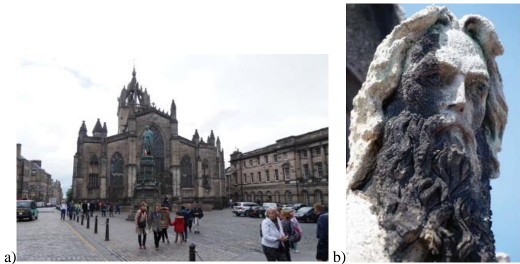
Figure 13. Crust pattern: a) black crust at the St Giles Cathedral, Edinburgh (Scotland, UK), b) detail of the black crust at the Naumburg Cathedral of St. Peter and St. Paul (Naumburg Cathedral, Germany, Image ICOMOS, 2009).
