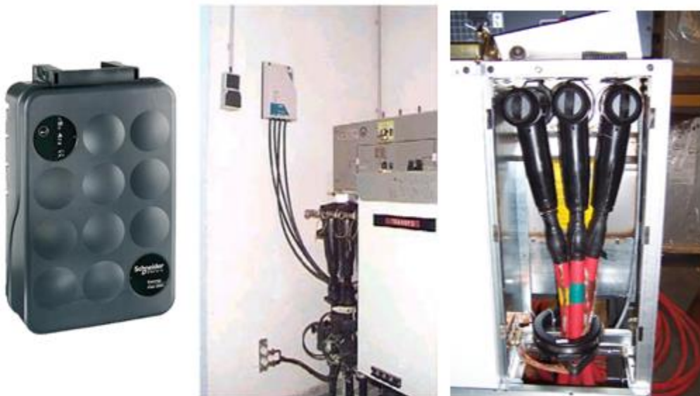
Figure 5.16 FPI in MV-LV substation, courtesy of Schneider Electric
