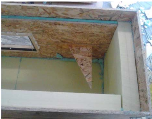
Fig. 4. Experimentel hut during its construction
