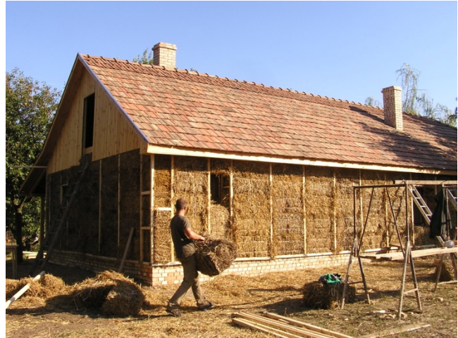
Fig. 5. Strawbale thermal insulation of an old adobe house
