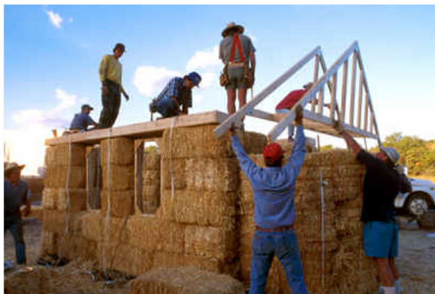
Fig. 1a Nebraska style (load-bearing) strawbale house during building
