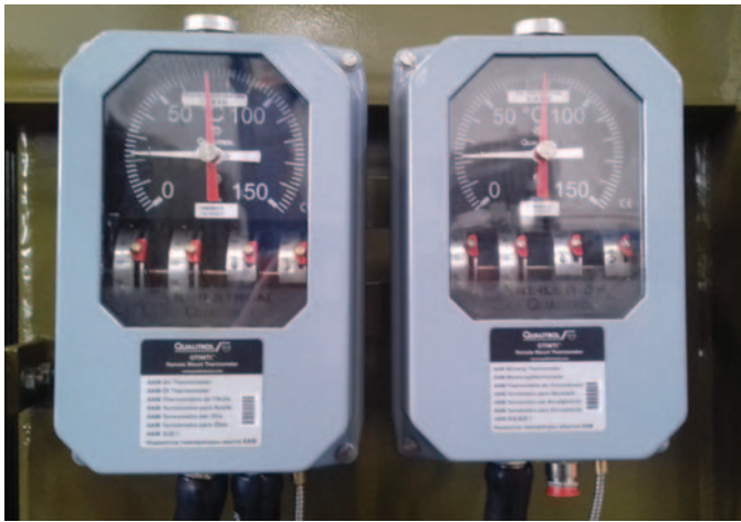
Figure 2: Typical top-oil and winding temperature indicators with alarm and trip contacts on a liquid-immersed transformer
