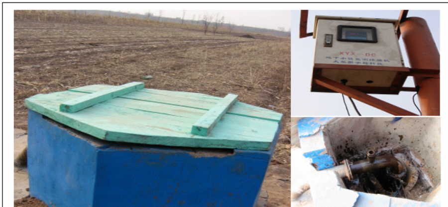
Figure 5: Model water saving district (left); Cash card apparatus (upper right) Embedded type irrigation pipe (lower right).
