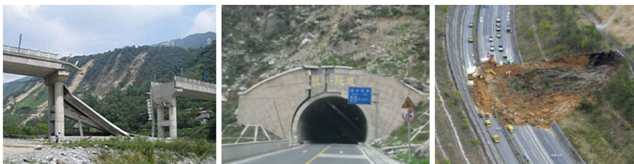
Fig. 3 Examples of traffic disruption due to key network component failures (bridges, tunnels and slopes)
