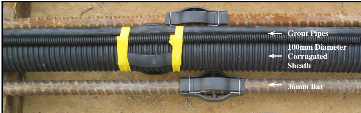
Plate 1 - Dywidag-Systems International soil nail double corrosion protection system
