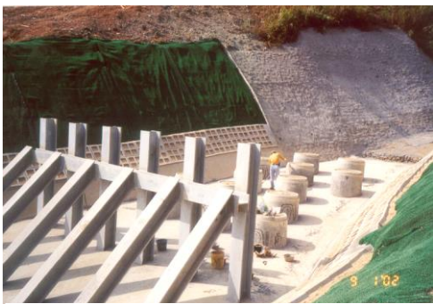
PLATE 5: View of debris flow depositional basin looking upslope
