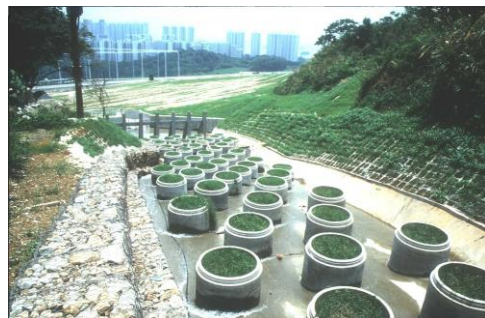
PLATE 6: Downslope view of debris flow depositional basin
