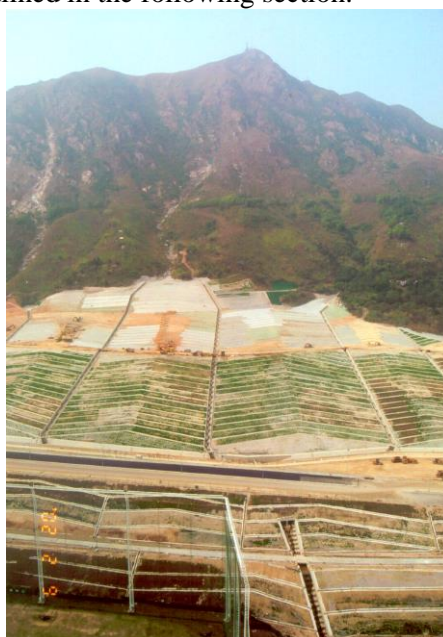
PLATE 4: Later Stages of Construction at Area 19, before construction of mitigation works
