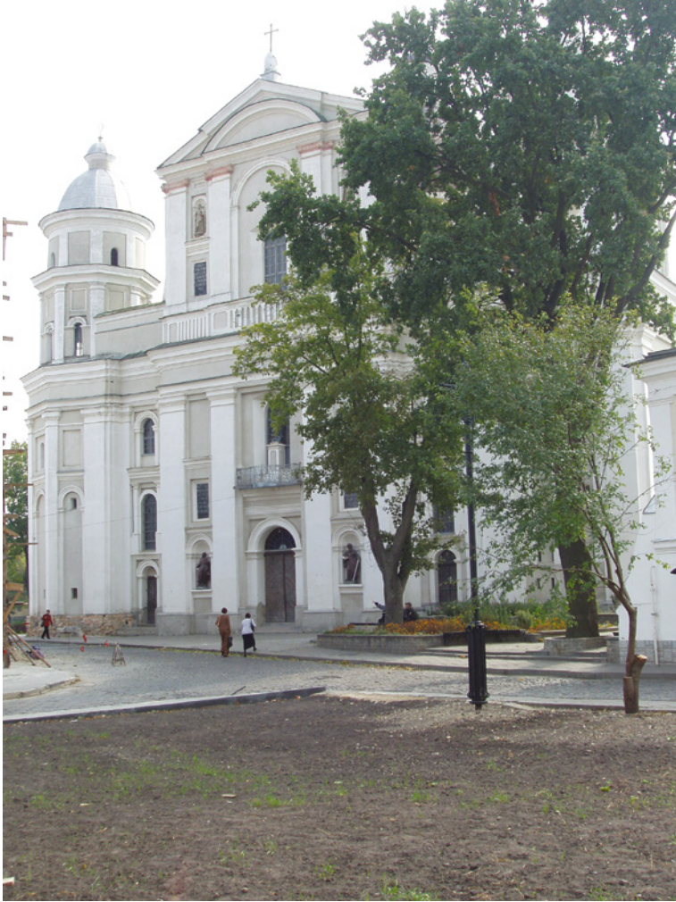
FIGURE 4 Façade of the Jesuit church in Lutsk (Łuck), built between 1616 and 1640, design by the Jesuit Giacomo Briano.
