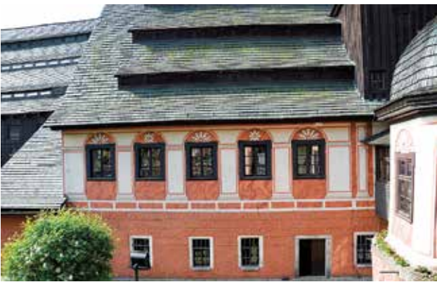
Photo 23. Part of the north-facing wall Photo by A. Fortuna-Marek
