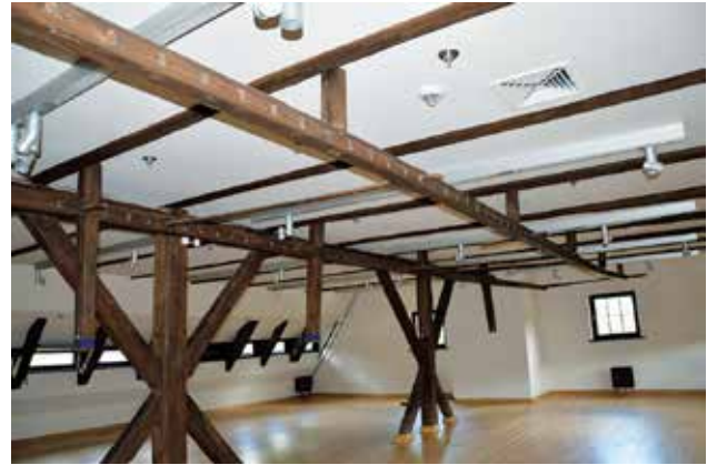
Photo 44. Drying house – interior after renovation works Photo by A. Fortuna-Marek
