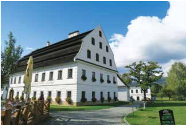
Photo 62. Velke Losiny. Paper mill. Photo A. Fortuna-Marek
