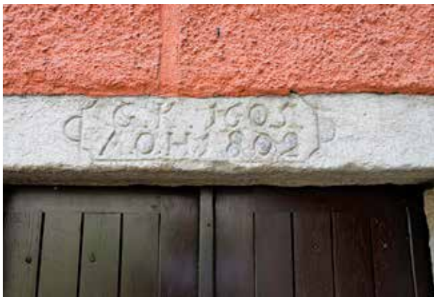
Photo 29. Inscription on the north portal Photo by A. Fortuna-Marek
