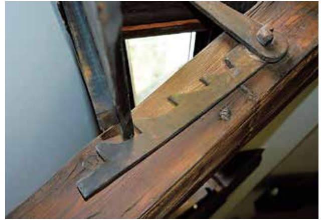
Photo 54. Flaps for regulating air flow Photo by A. Fortuna-Marek
