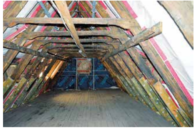
Photo 51. Roof framework of the paper mill building Photo by A. Fortuna-Marek
