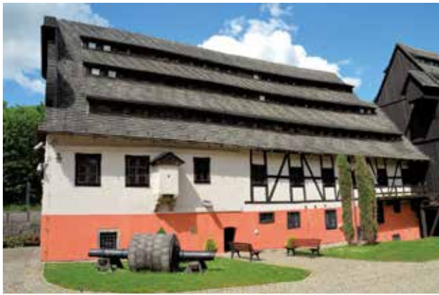
Photo 27. Paper mill wall facing south Photo by A. Fortuna-Marek
