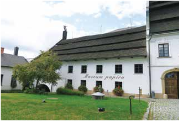
Photo 61. Velke Losiny. Paper mill. Photo A. Fortuna-Marek
