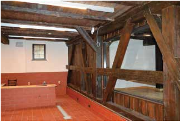
Photo 43. Drying house – interior after renovation works Photo A. Fortuna-Marek
