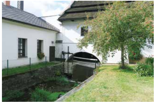
Photo 64. Velke Losiny. Paper mill. Photo A. Fortuna-Marek
