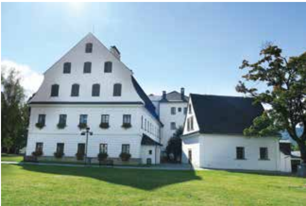
Photo 63. Velke Losiny. Paper mill. Photo A. Fortuna-Marek
