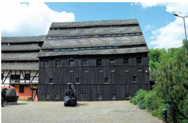
Photo 31. South-facing wall of the drying house Photo by A. Fortuna-Marek
