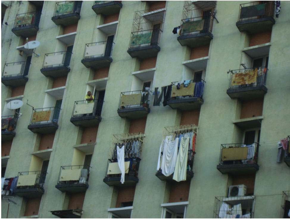
High-Rise Flats Source: J. Crush
