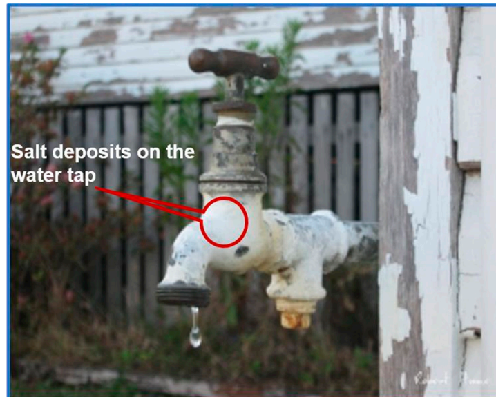
Figure 1. A picture showing public water tap with a salt deposit in Limpopo Province, South Africa [5].
