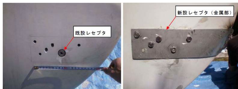
Figure 3.32: Tip receptor retrofit. Initially disk receptors were installed. Retrofit to band type receptors resulted in significant lightning performance improvements (Figure adapted from [9]).
