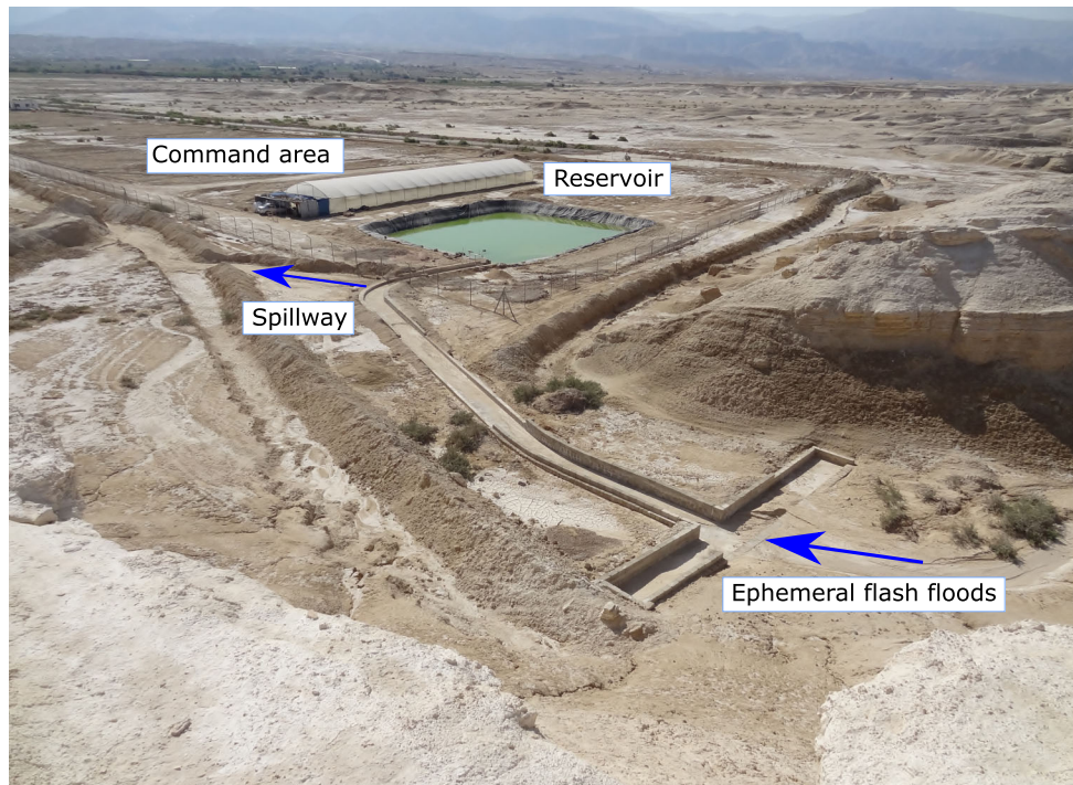
Fig. 1 Panoramic view of irrigation scheme with reservoir for harvesting flash floods
