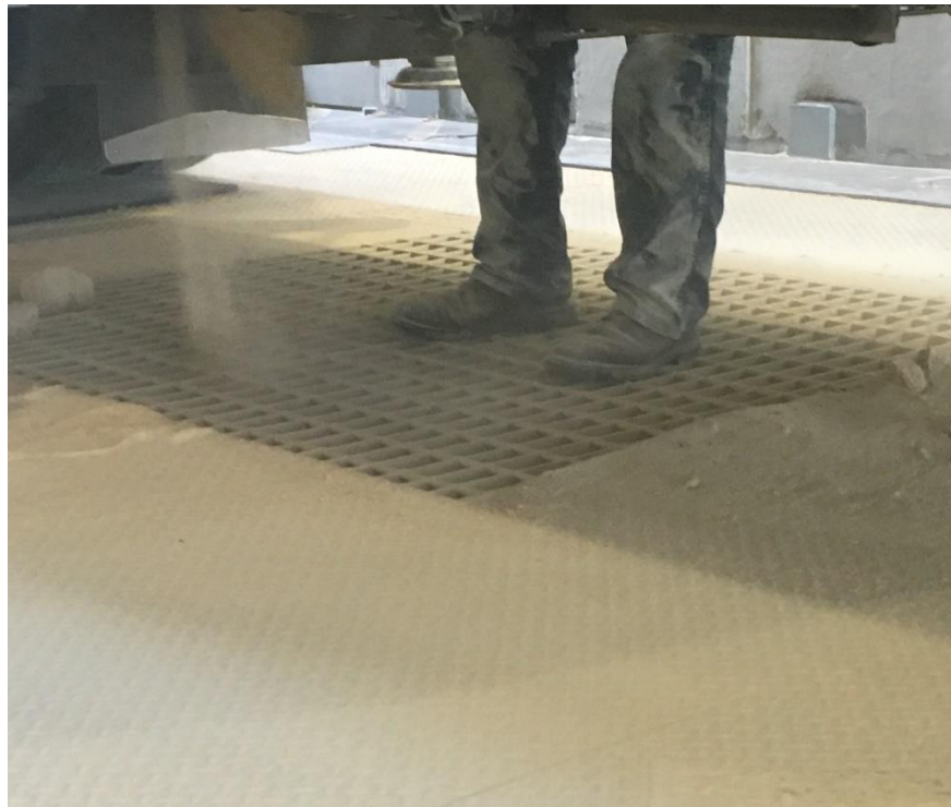
Figure A-8. Receiving area floor
