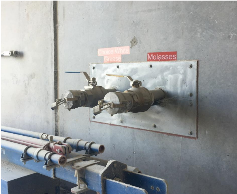
Figure A-2. Fat intake inlet
