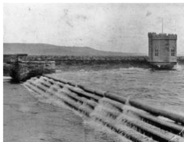
Langsett Reservoir Post Construction
