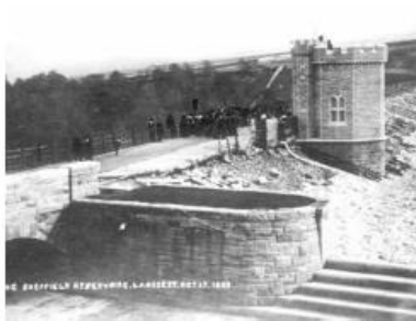
Langsett Reservoir During Construction
