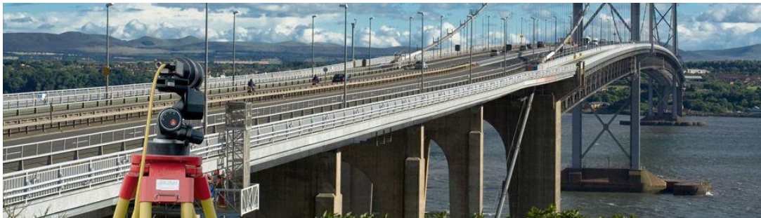
Figure 2-6. High speed camera for highway bridge monitoring (iMetrum 2017)
