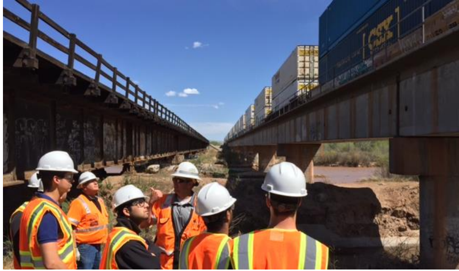
Figure 2-1. Visual inspection of railroad bridges.
