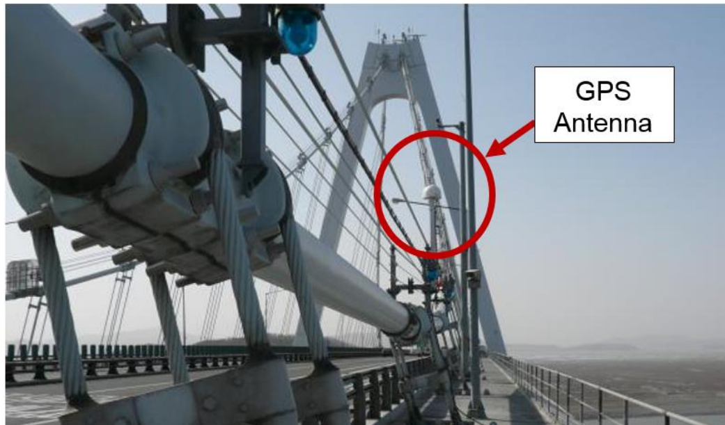
Figure 2-4. GPS for bridge displacement measurement (Carnenbroeck 2015)
