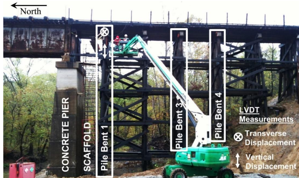
Figure 2-2. Transverse bridge displacement using a LVDT (Moreu et al. 2015a)
