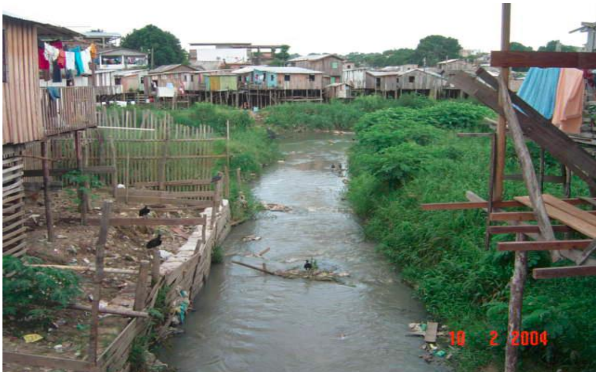
Figure: 2 - Precarious housing conditions in Brazil
