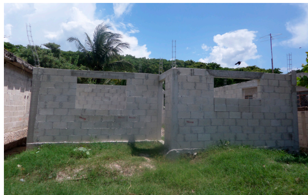
Figure 4. Typical confined concrete masonry construction in Yucatan communities (photo: L. Bank).
