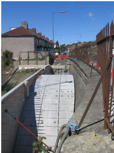
c) Ready for backfilling
