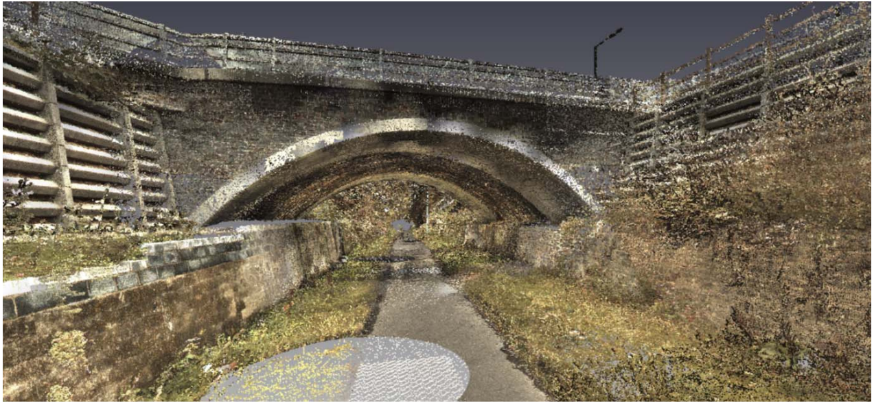
Figure 4 Point cloud laser scan of bridge from cycleway
