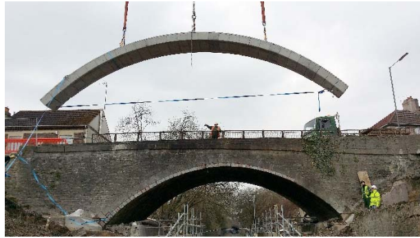
b) Lowering first FlexiArch unit into position
