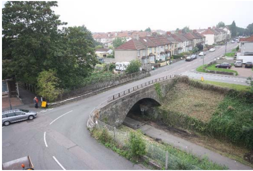
a) Original bridge/junction
