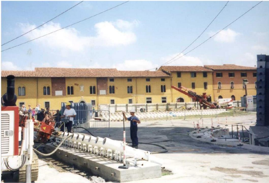
Figure 2 Boreholes for final works of under-excavation
