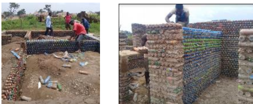
Figure 8: Plastic bottle Wall construction
