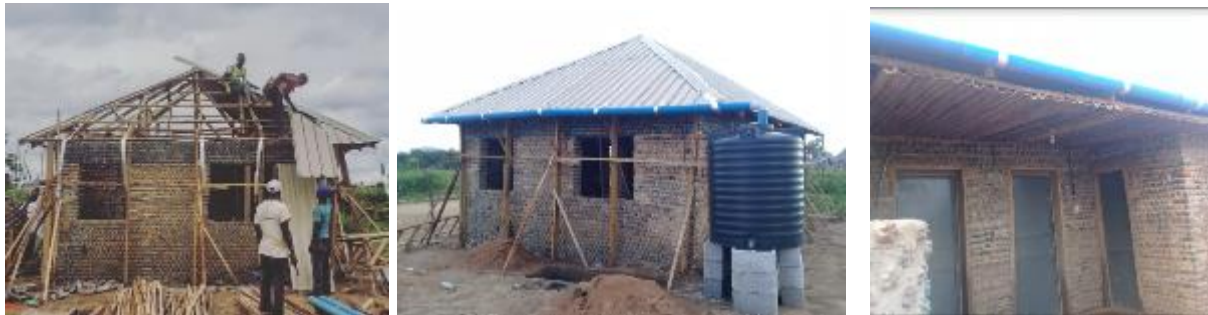
Figure 9: Roof Construction with rainwater harvesting
