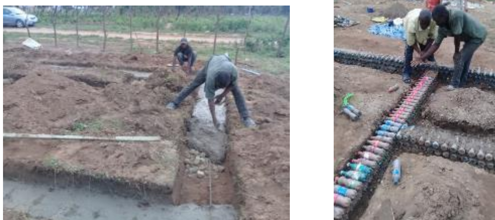
Figure 7: Foundation works for prototype
