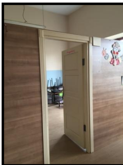
Figure 14. An example of classrooms were each separated into two smaller classrooms by a board in Turkish special education school
