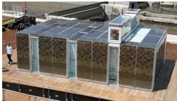
Fig. 2.22 The PVT prototype tested on a Solar Decathlon house (Eicker and Dalibard 2011). Calise et al. (2016) proposed and simulated a novel poly-generation system which combined PVT collectors, a heat pump and an adsorption chiller to supply electricity, domestic hot water, and indoor space heating and cooling. This system could use 49% of the total solar energy with a yearly COP over 4 for cooling and 5.5 for heating, respectively. The thermos-economic optimisation for the system can reduce the simple pay-back period from over 16 years to around 14.5 years.
