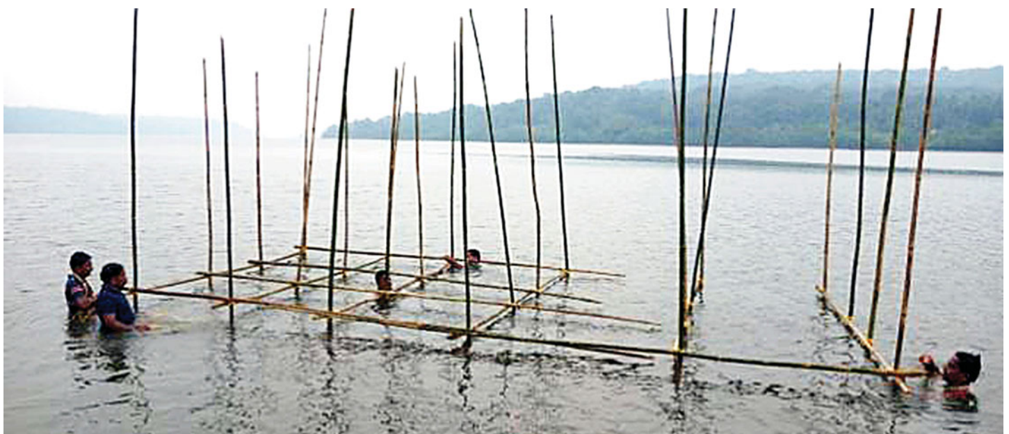
Construction of a rack at Wadatar
