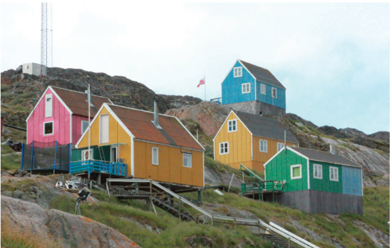
Figure 10.1 Typical colorful, one-family gable-roofed housing in Sarfannguaq, Greenland (photo by Tove Lading).
