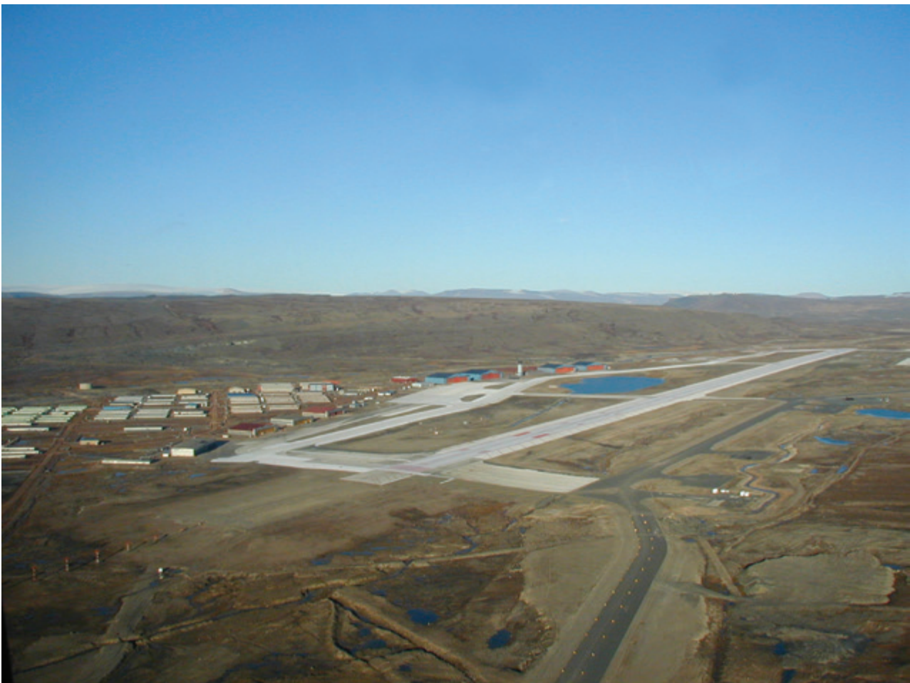
Figure 10.15 Runway, Thule Air Base: 3000 m of flexible asphalt pavement (photo by Kevin Bjella).
