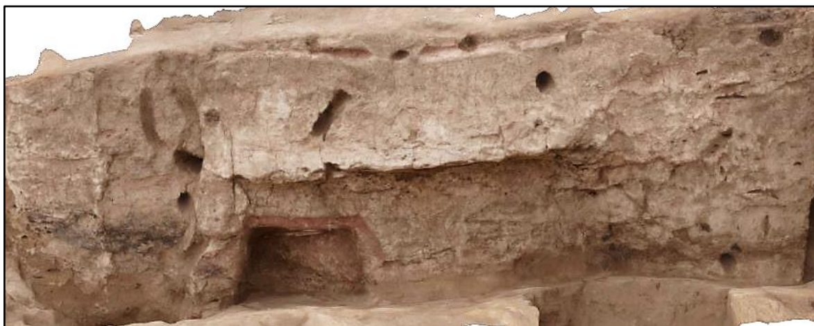
Figure 5.8 View of South wall of Space 87. Orthophoto by M. Perlińska.
