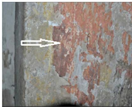
Figure 9: Details of the paint with visible evidence of the original layer (white arrow).
