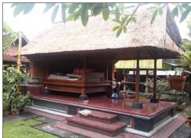
Fig. 1 Bale “Sakenem” Building
